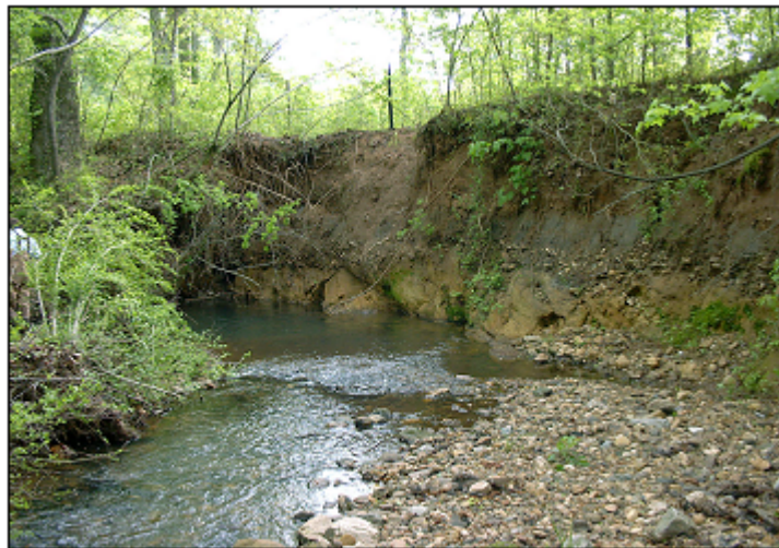
Figure 1.1-6 Example of Stream Channel Bank Erosion
