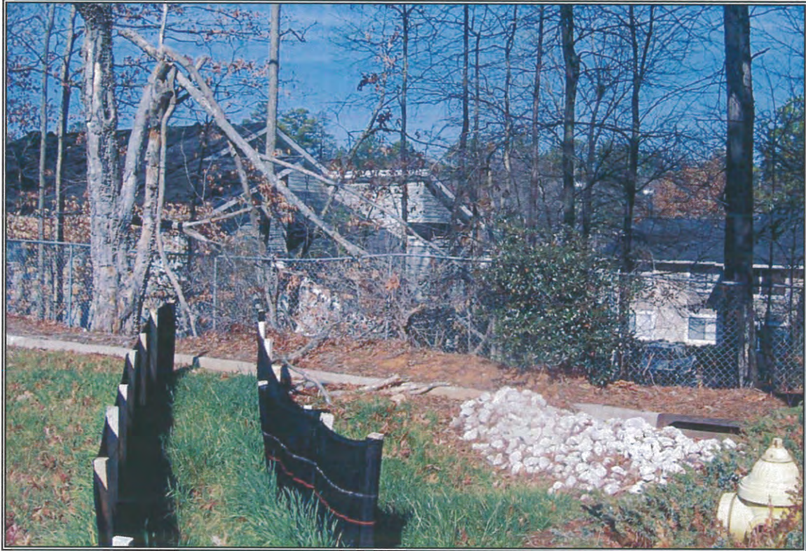
PHOTO 1 Drains and erosion control at the 4575 parcel
