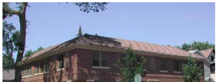
Roof Materials: Ceramic Tile
