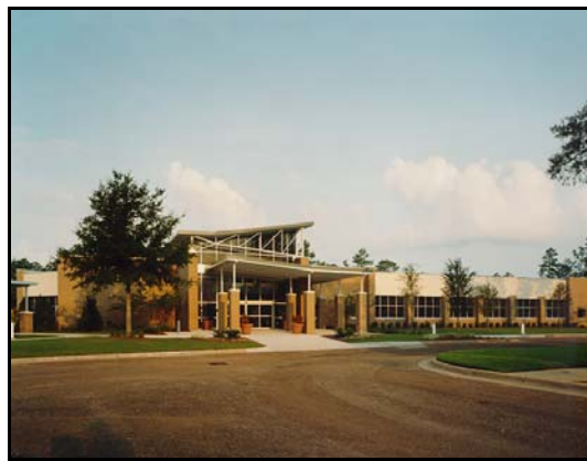
Exterior of Niceville Library
