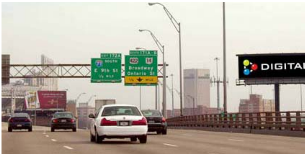
Figure 1. Proximity of DBB #3 to an interchange. This same DBB is shown in Figure 2-8, p. 16, of the Tantala study. It is also Site # 22 from the Lee, et al (2007) study, discussed in detail below.
