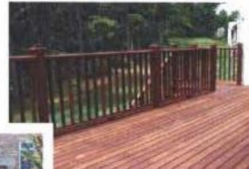
Wood Deck & Railing with Pickets at 4"oc
