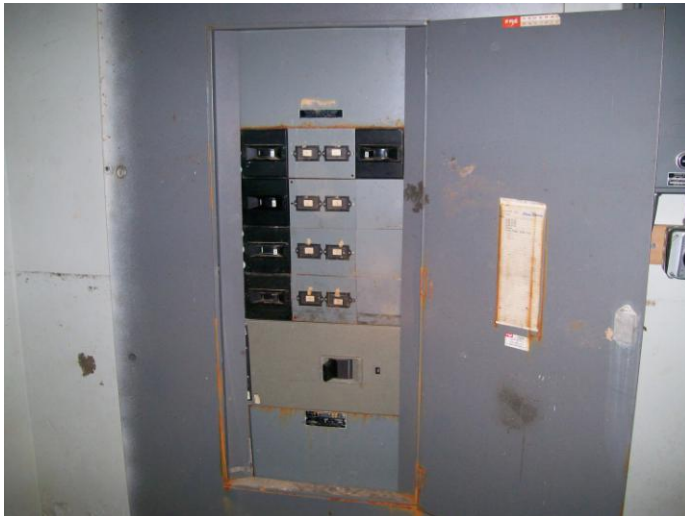
Water Damage at Main Distribution Panel “PP-L”
