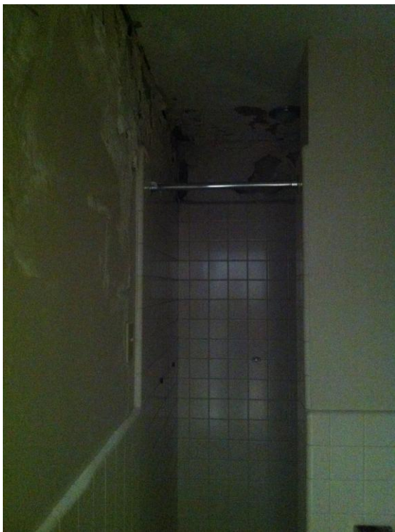
Damaged Wall at Restroom/Shower
