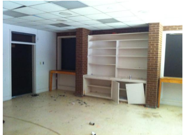
Damaged Flooring & Millwork
