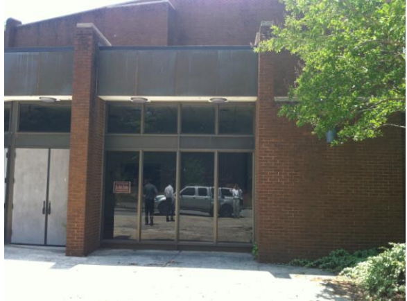
Original Glazing in Aluminum Storefront
