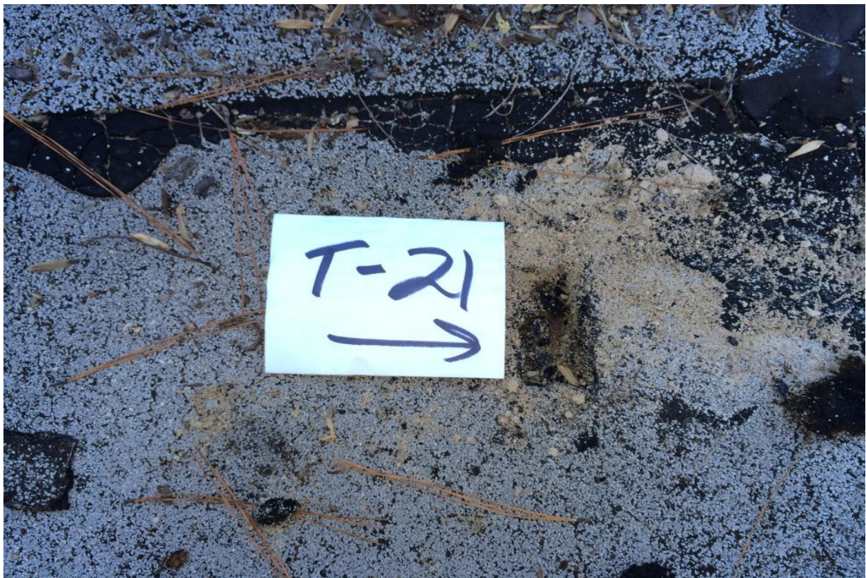
Plate 70: Laboratory analyses did not detect asbestos minerals within asphalt roof sample TS-21 collected from the Theatre Building roof.
