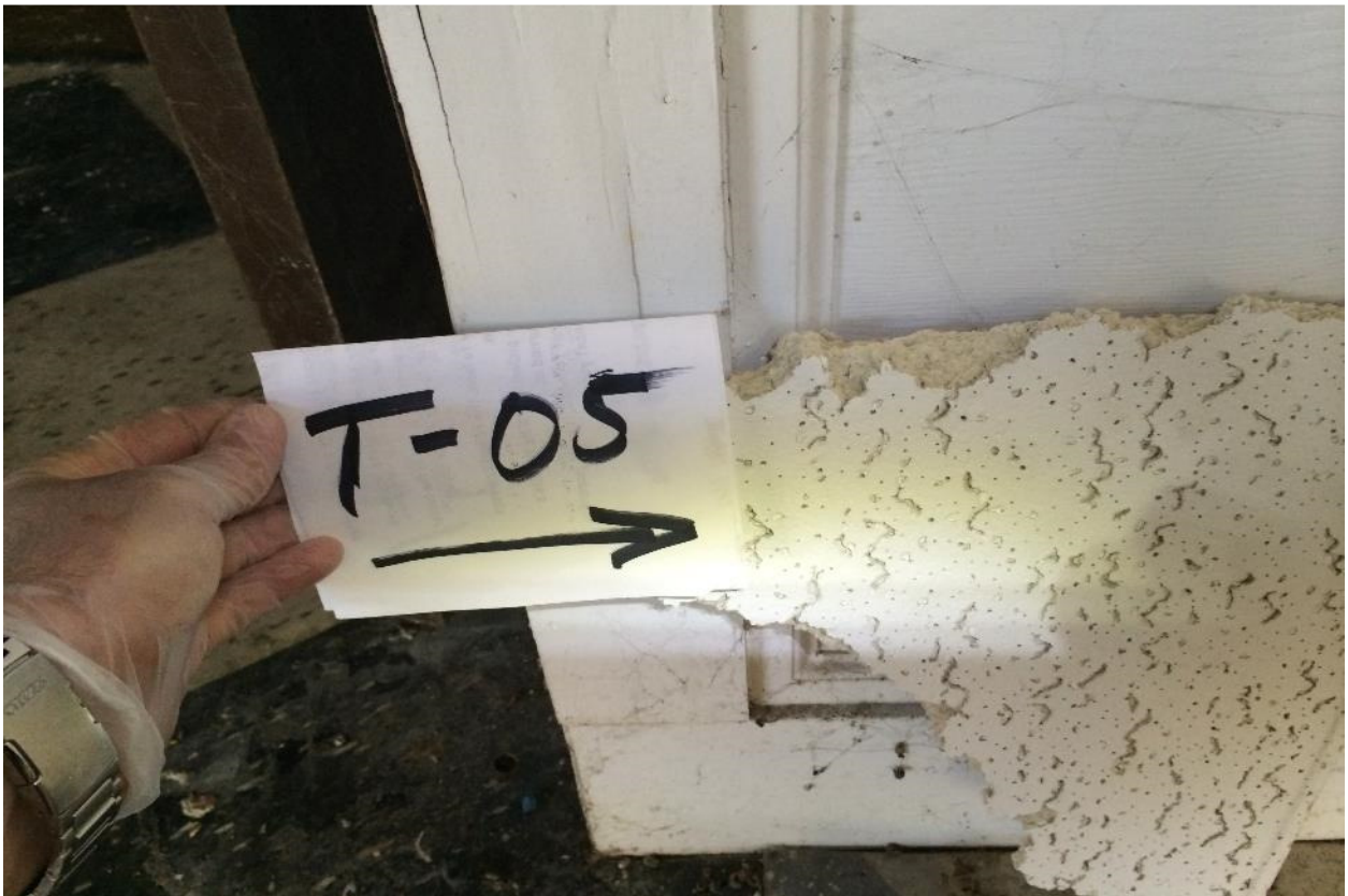
Plate 56: Laboratory analyses detected 2% chrysotile asbestos within suspended ceiling tile sample TS-05 collected from the Theatre Building lobby area.
