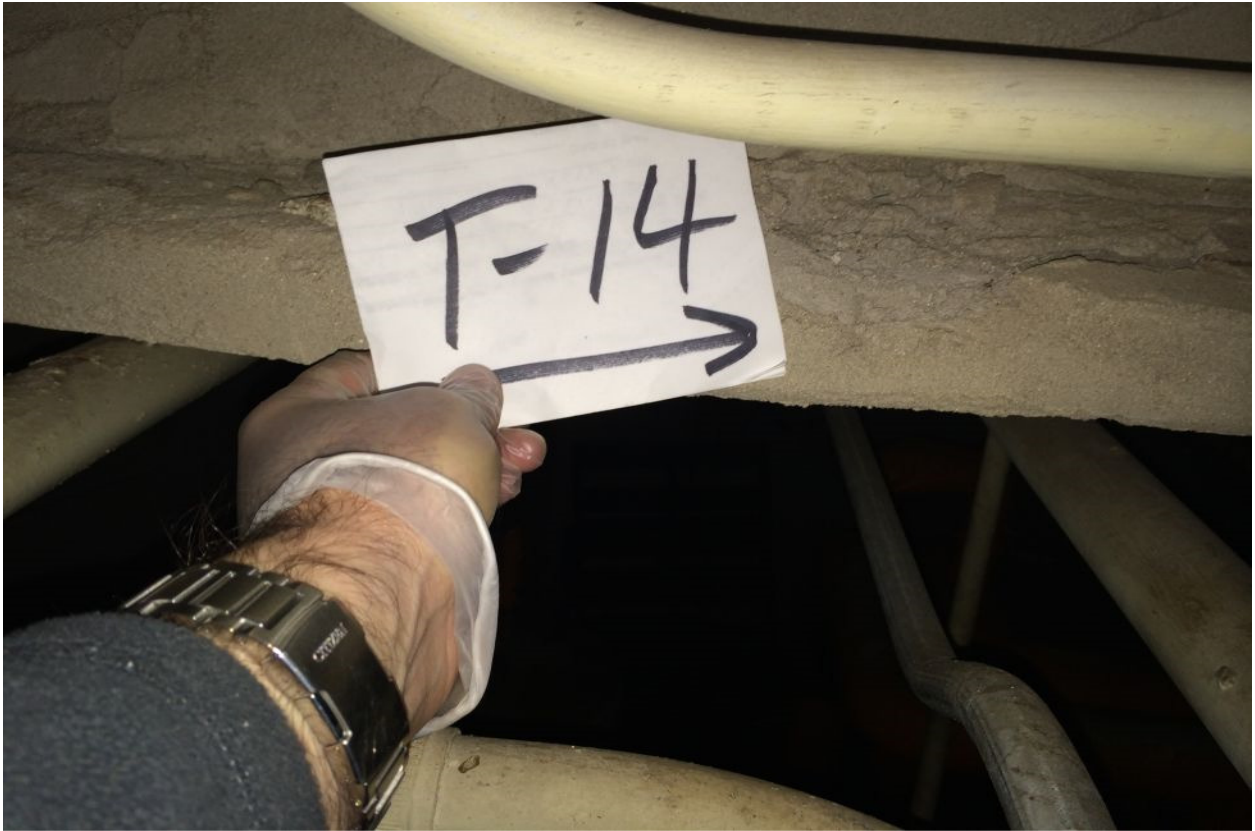
Plate 65: Laboratory analyses detected 20% chrysotile asbestos within spray on surfacing material sample TS-14 collected from the Theatre Building basement structural steel.
