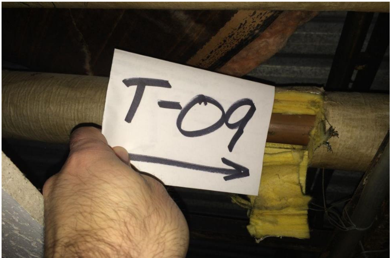
Plate 60: Laboratory analyses did not detect asbestos minerals within plumbing insulation sample TS-09 collected from the Theatre Building lobby ceiling.
