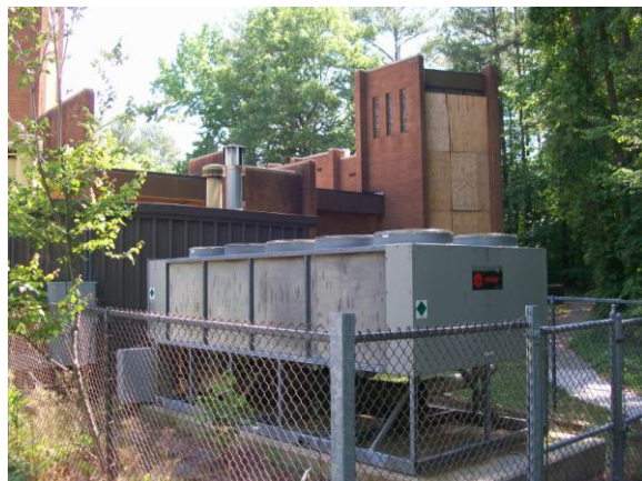
Chiller at Rear of Facility
