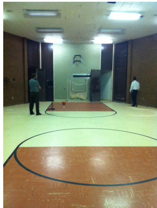
Damaged Walls at Recreation Room
