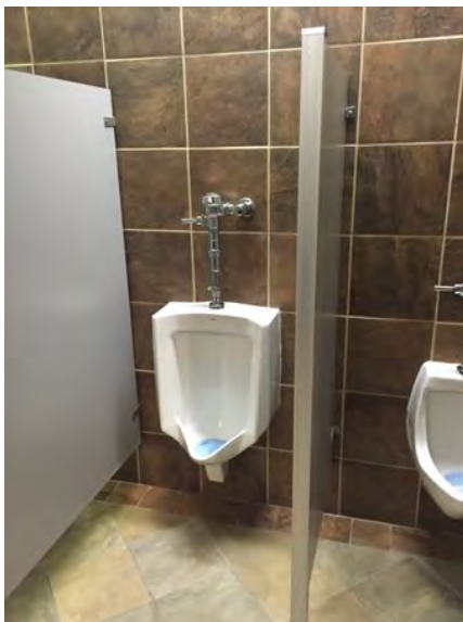
Standard Flush Valves
