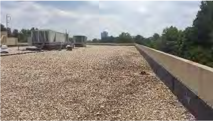
Loose Laid Ballast EDPM Membrane at Perimeter: - or open at base flashings.
