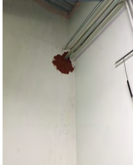
Fire sealing missing
