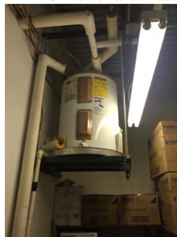
Electric Water Heater
