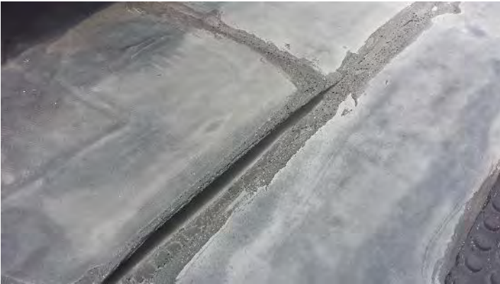
Repairs at base flashing done with improper materials
