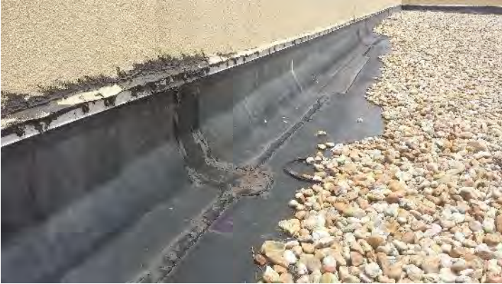
Many repairs observed were done with improper material. As a result, these repairs are failing.
