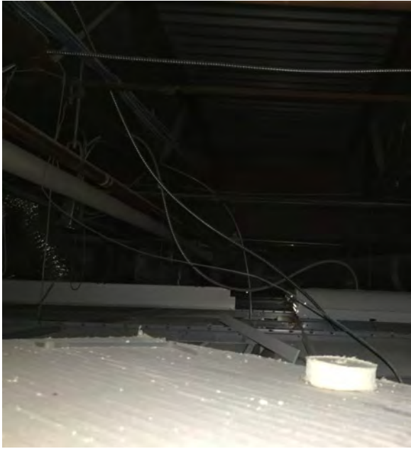
MC Cable above ceiling
