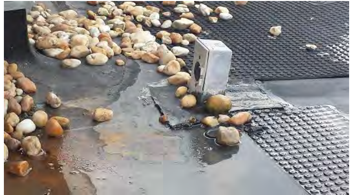
Standing water was present at various locations at HVAC flashing.
