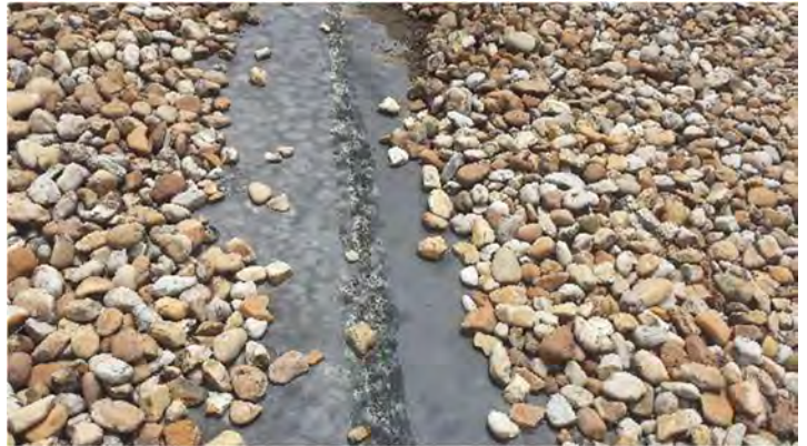
Field lap sealants and adhesives are deteriorating.
