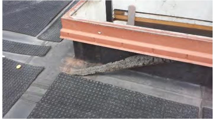
Foam material termination at roof hatch is loose and deteriorated.
