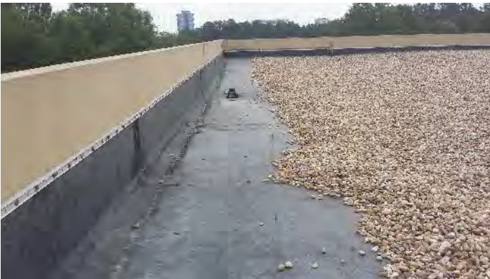
Insufficient ballast was observed in localized locations.
