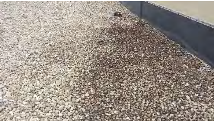
Evidence of red algae growth, in the ballast, at some locations. This may be a result of the roof drain not set low enough to function properly.
