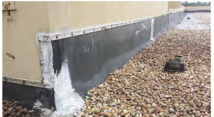
Termination bar was observed to have multiple inconsistent types of sealants.
