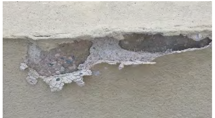
Moisture intrusion was observed between cast parapet wall and cementitious coating on south elevation.
