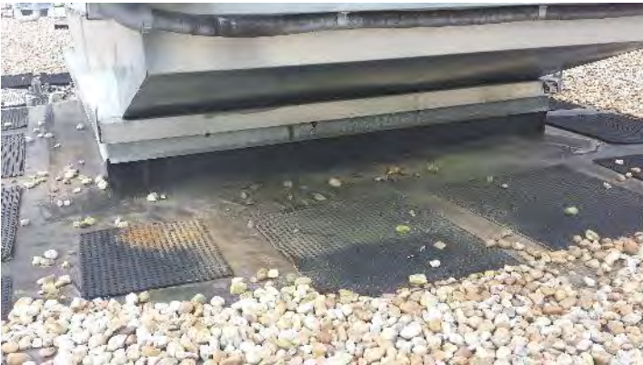
Deterioration of membrane integrity, likely caused by petroleum based fluid spill, was observed at an HVAC
