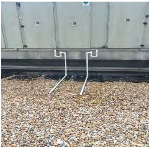
RTU Condensate Piping
