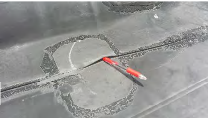
Membrane seam lap sealant is deteriorated or open at base flashings.
