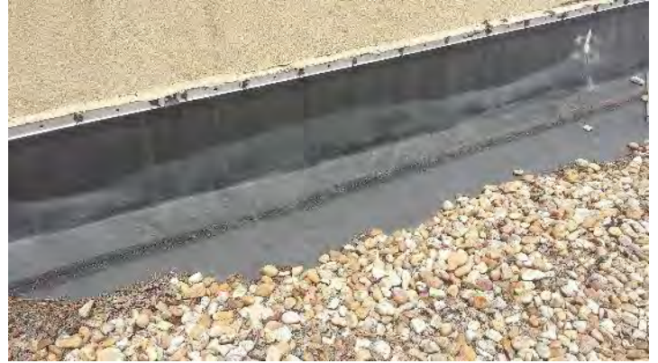
Perimeter base flashing display bridging or shrinkage at most of the assembly.
