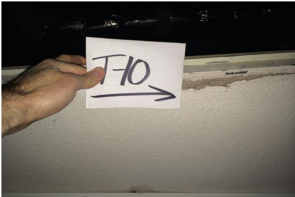
Plate 61: Laboratory analyses detected 20% chrysotile asbestos within spray on surfacing material sample TS-10 collected from the Theatre Building upstairs projection room ceiling.
