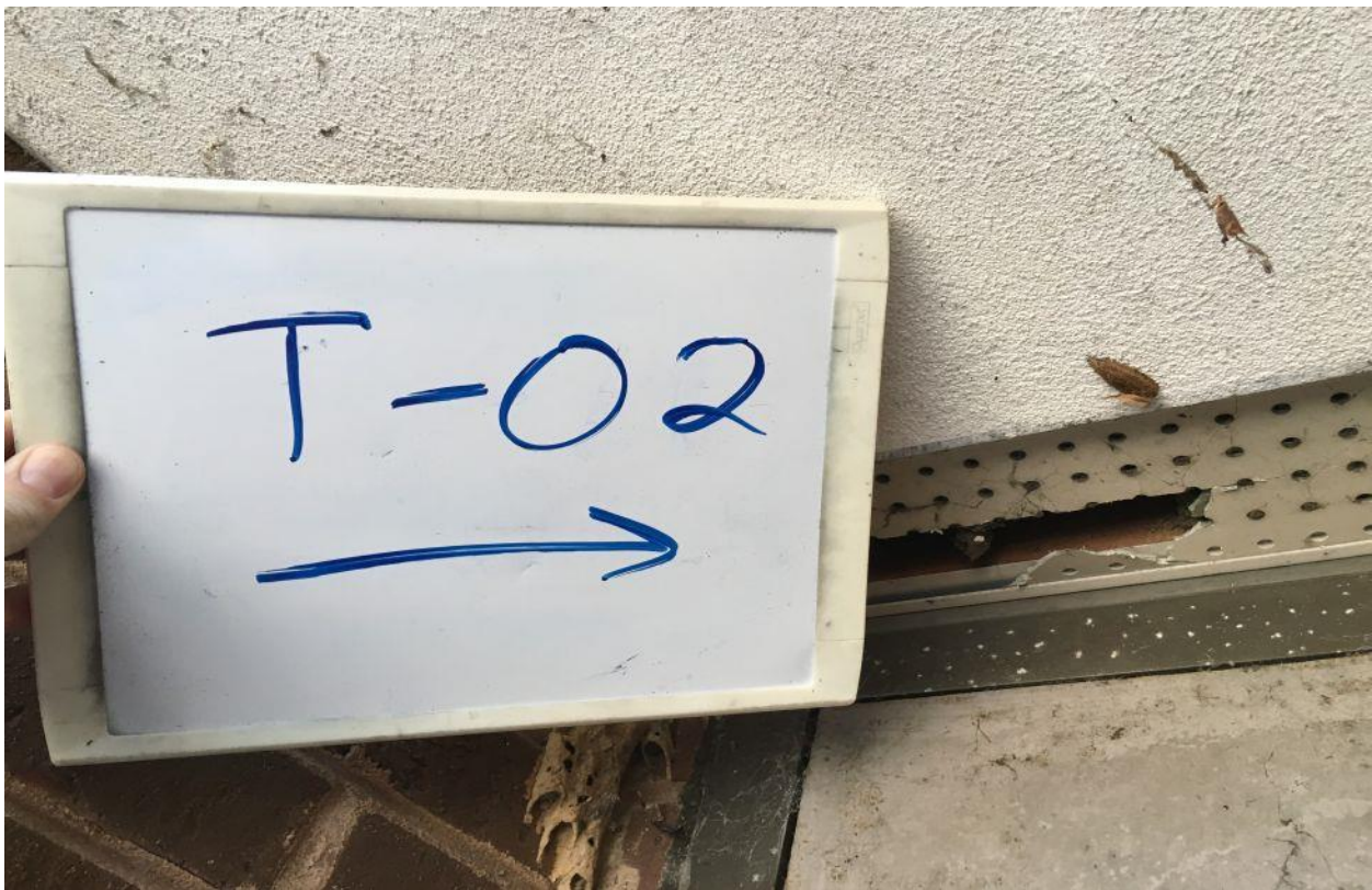
Plate 2: Laboratory analyses detected 20% chrysotile asbestos within transite ceiling tile sample T-02 collected from the north side lobby entrance overhang of the Theatre Building.
