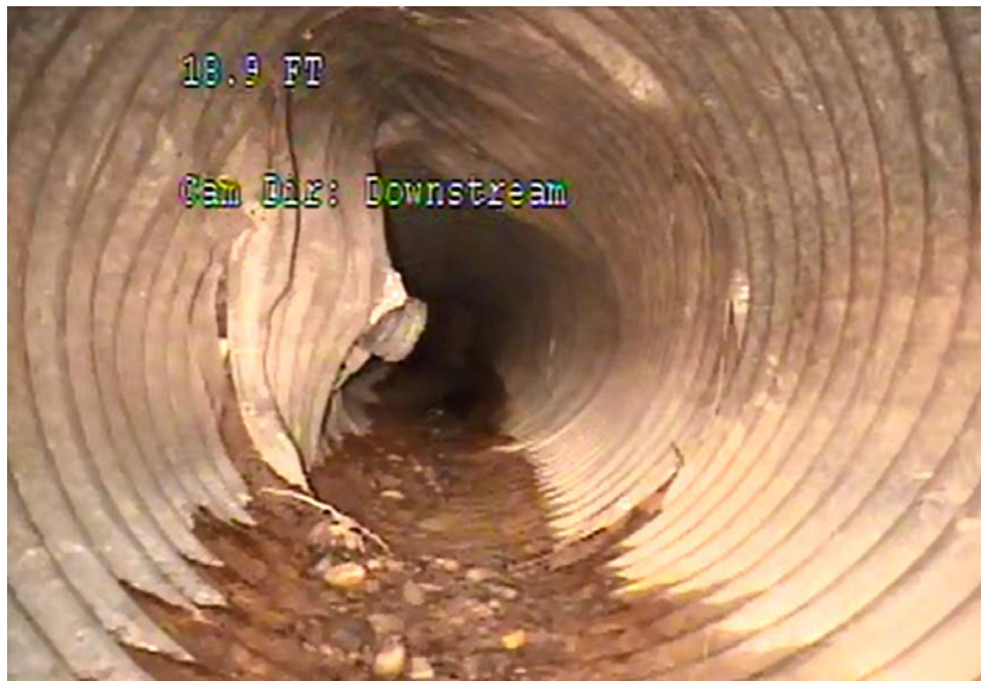
Required Point Repair between 5028 and 5036 Vermack Road
