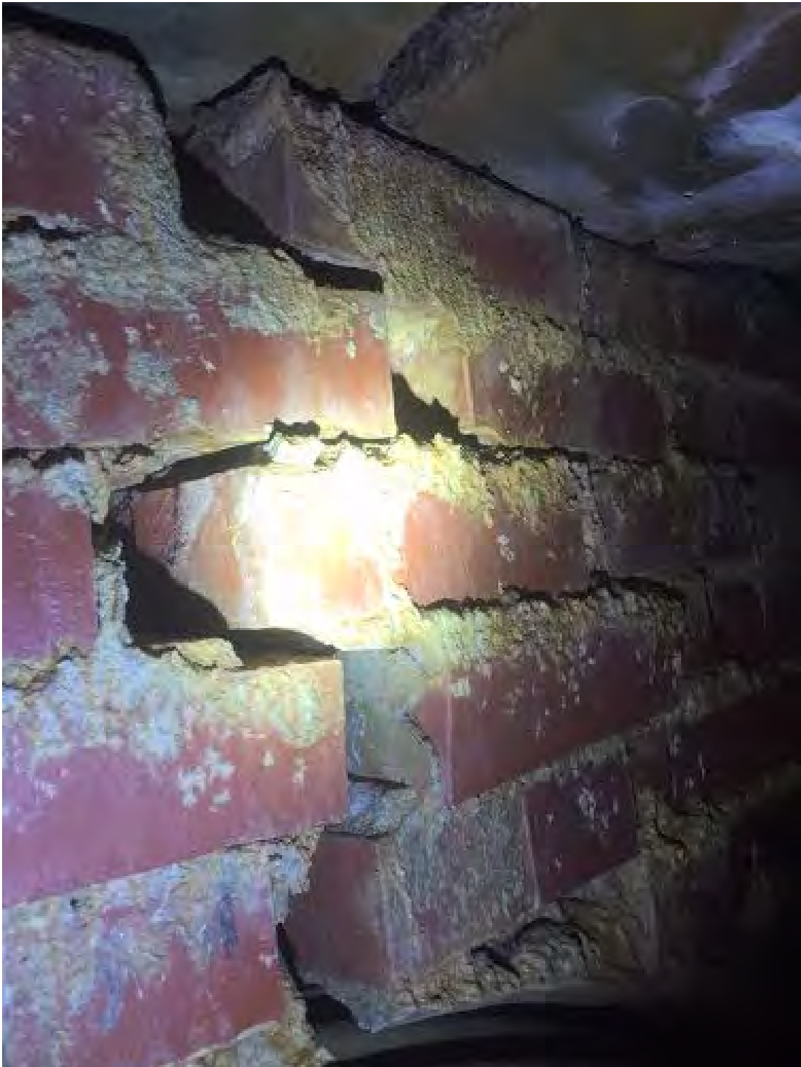
Large cracks in failing junction box
