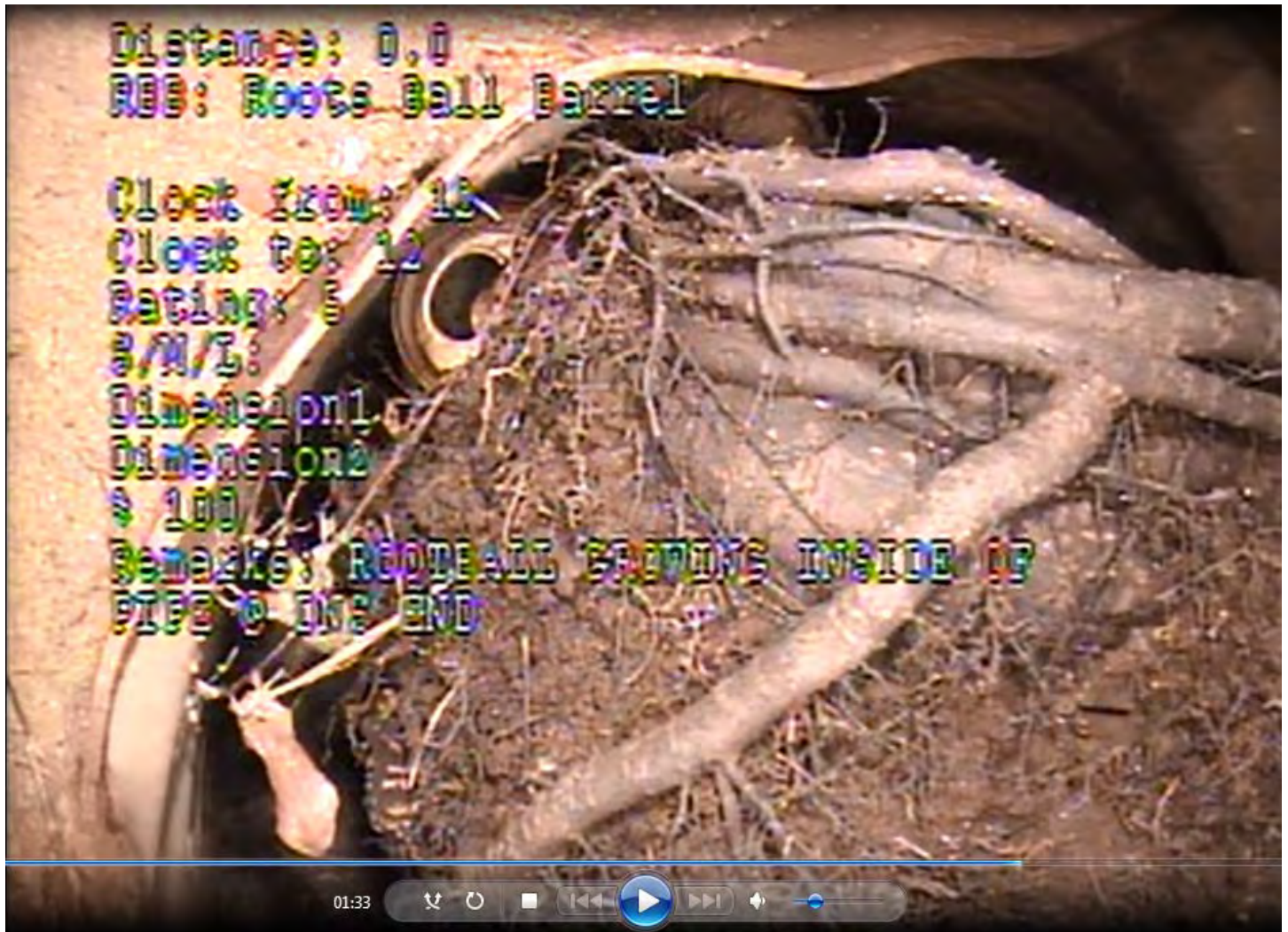
Root ball causing flow restriction and sinkhole (has been removed)
