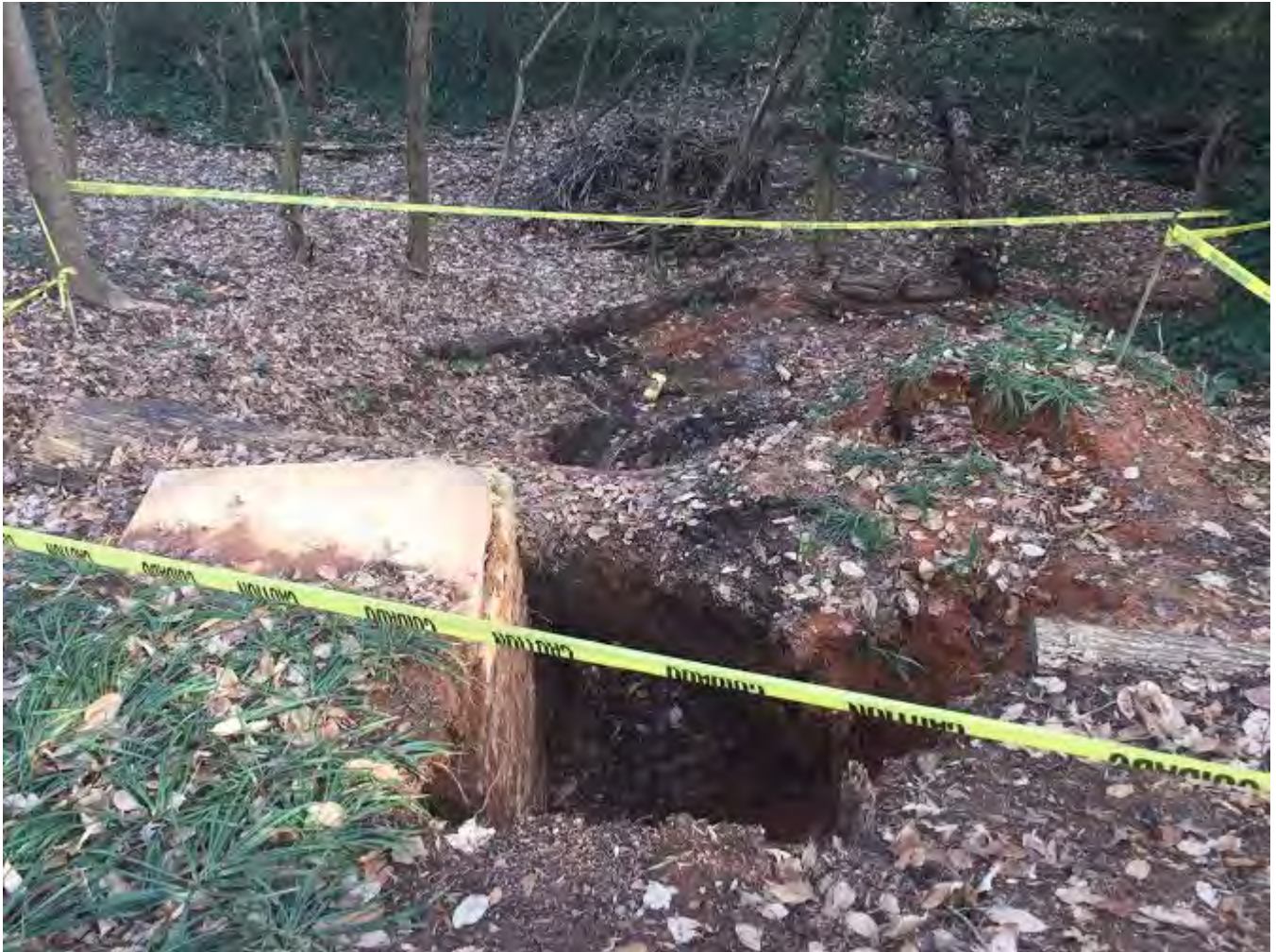
Large sinkhole resulting from a downstream culvert failure
