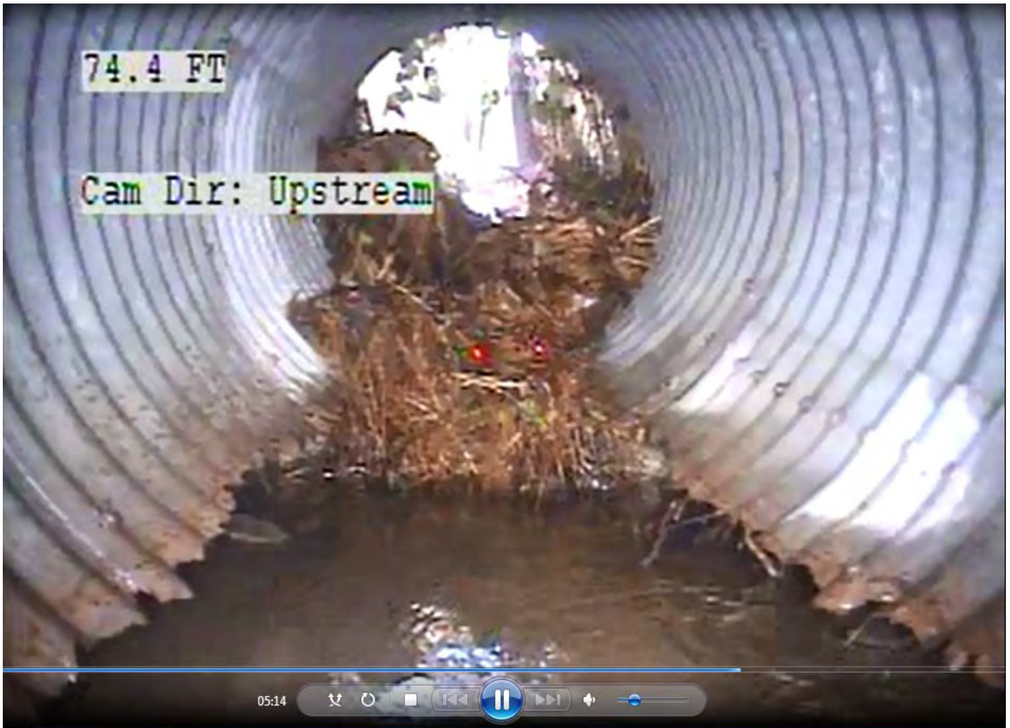
Failing portion of upstream culvert
