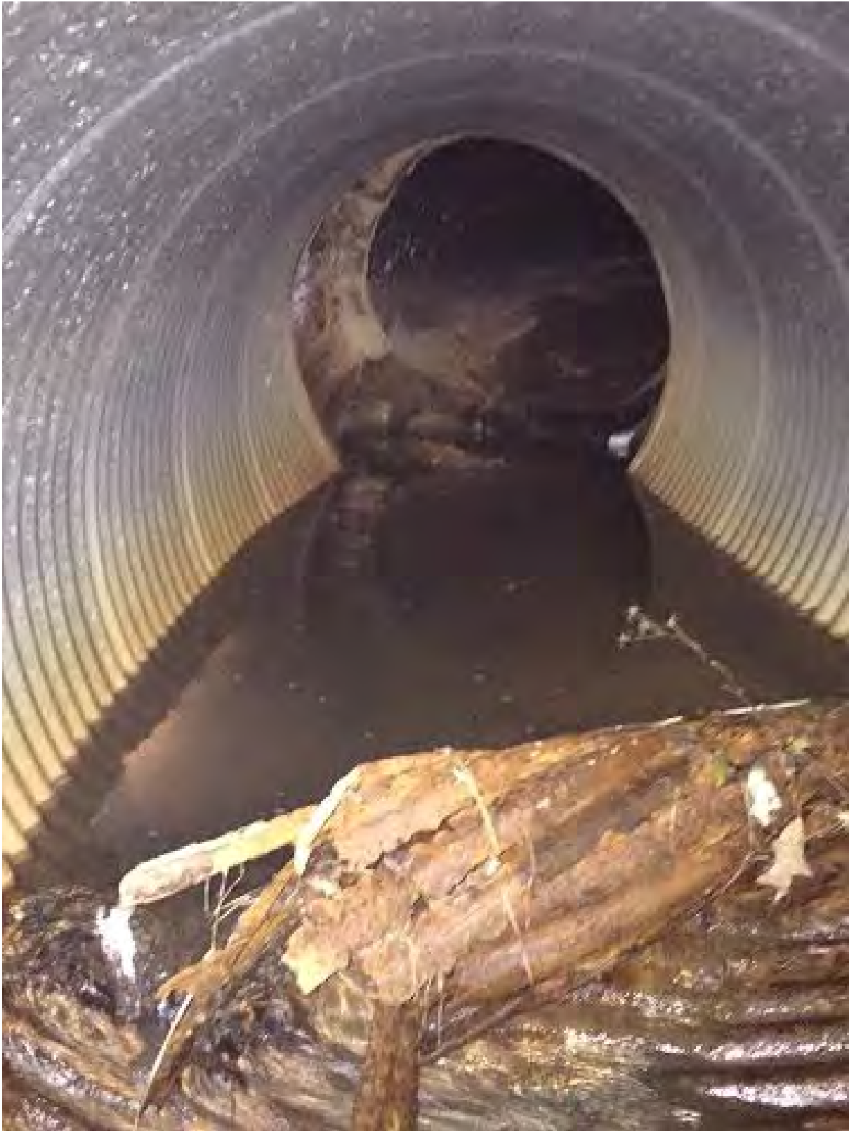
Failed Pipe Segment under Sinkhole
