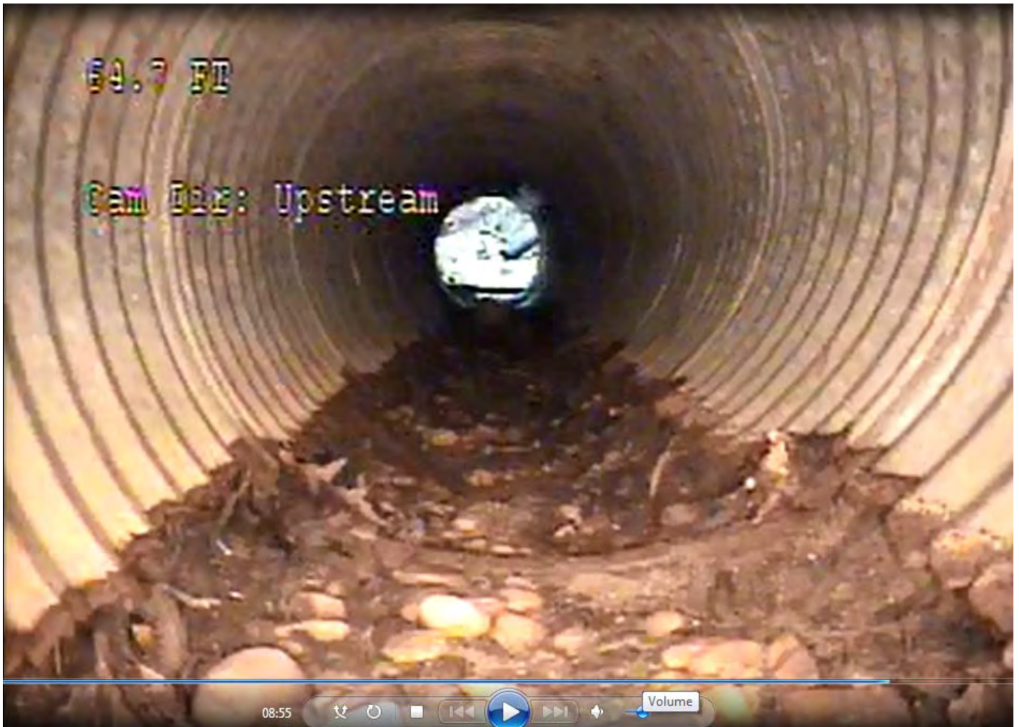
Deteriorated portion of CMP
