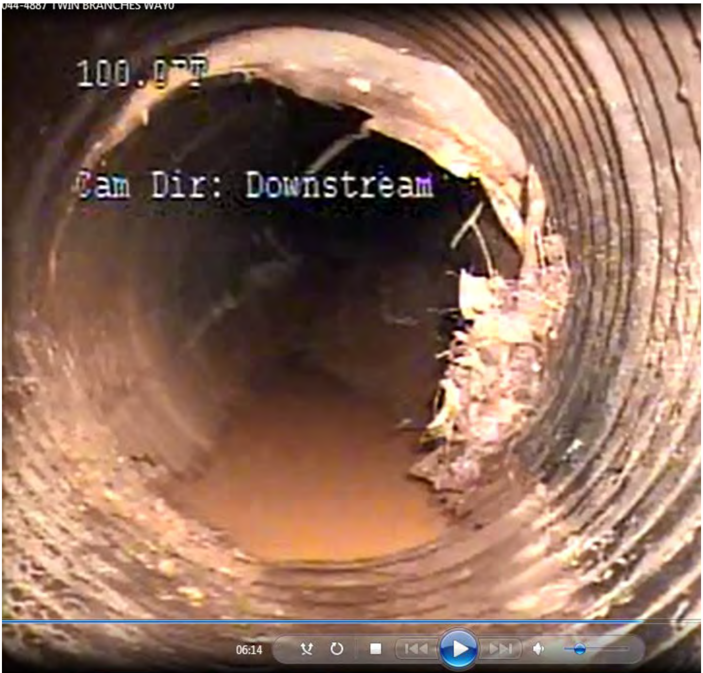
Culvert failure requiring internal point repairs prior to CIPP lining
