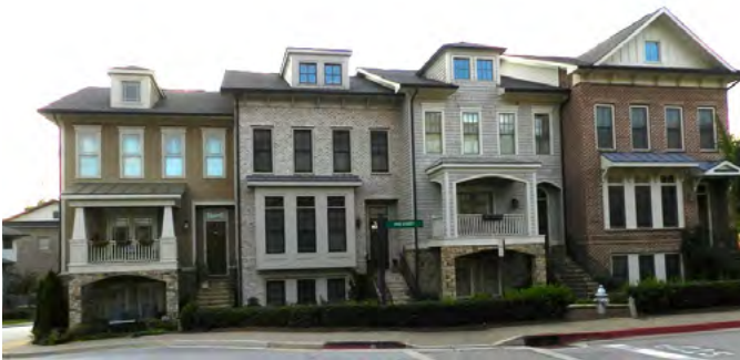
Figure 27-98-34 Examples of Ground Story along Slope.
