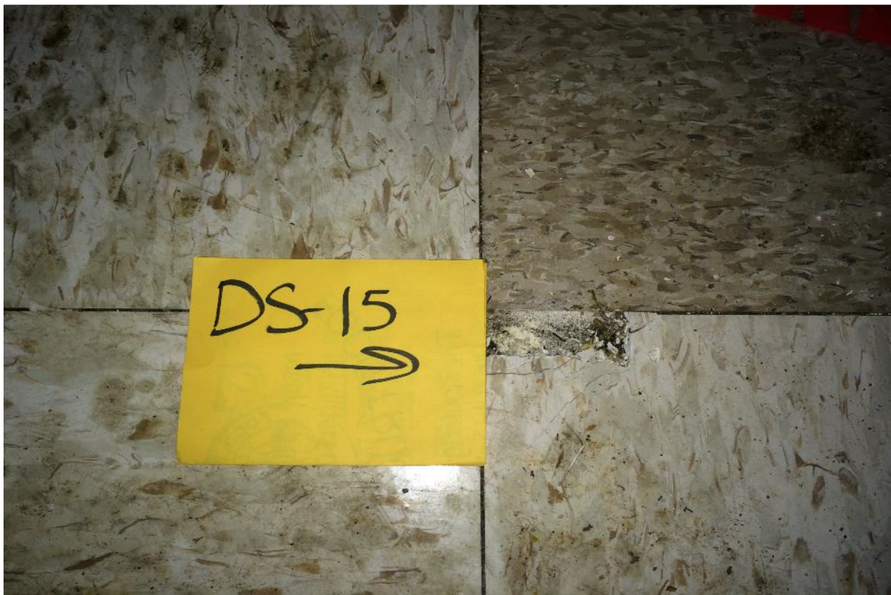
Plate 40: Laboratory analyses did not detect asbestos minerals within the tan and white floor tile or mastic sample DS-15 collected from the Dormitory Building downstairs hallways.
