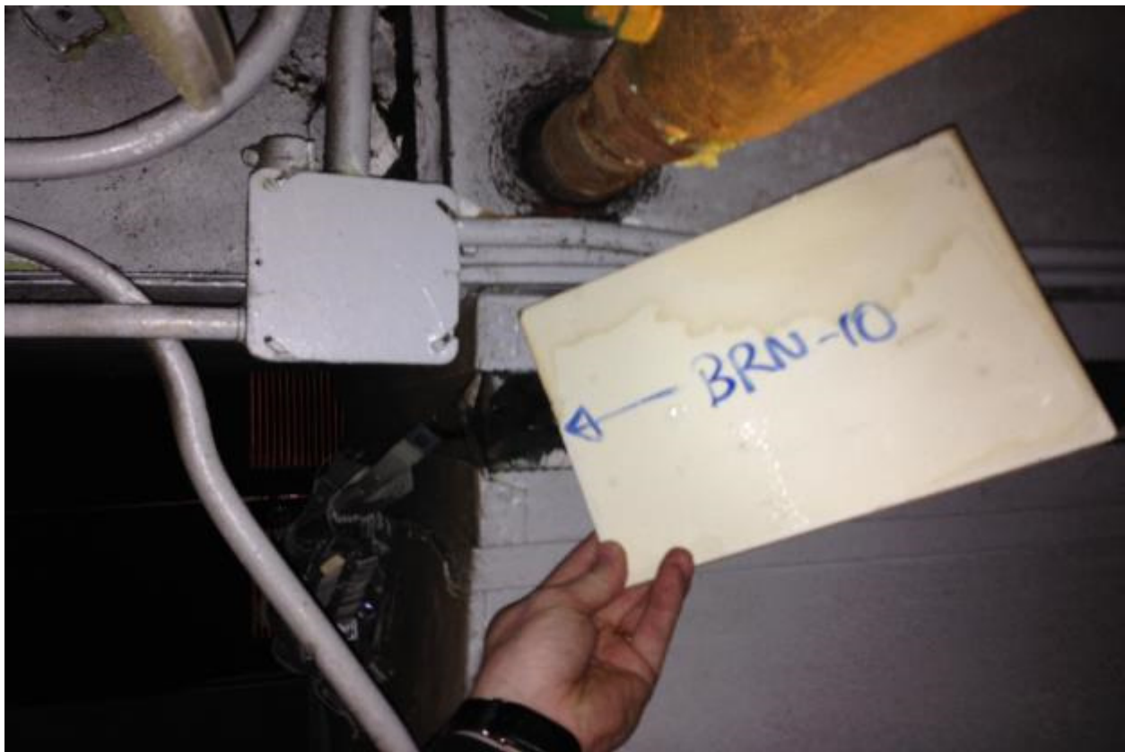
Plate 10: Laboratory analyses did not detect asbestos minerals within HVAC gasket sample BRN-10 collected from the North Administrative Building mechanical room.
