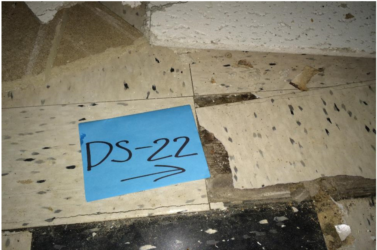
Plate 47: Laboratory analyses did not detect asbestos minerals within the black and white floor tile or mastic sample DS-22 collected from the Dormitory Building downstairs training room.
