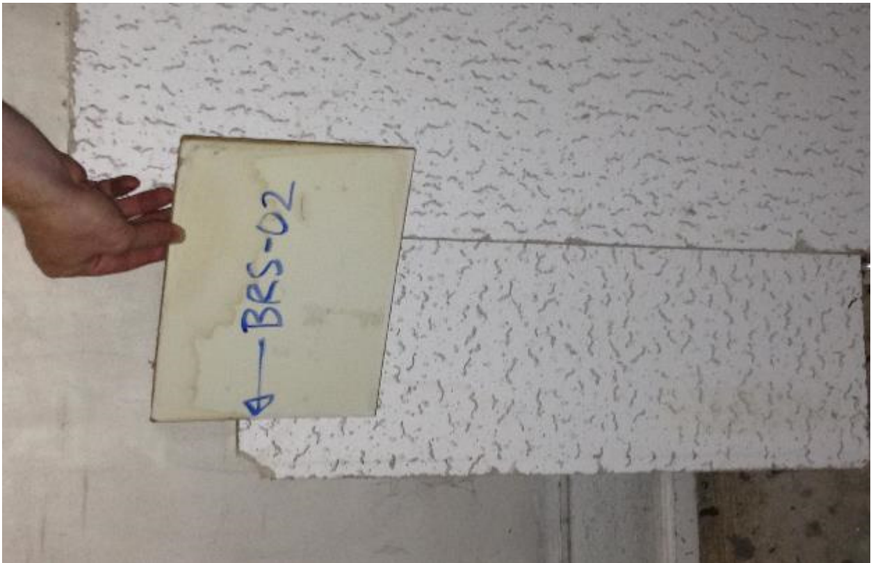
Plate 2: Laboratory analyses did not detect asbestos minerals within suspended ceiling tile sample BRS-02 collected from the South Administrative Building west room.
