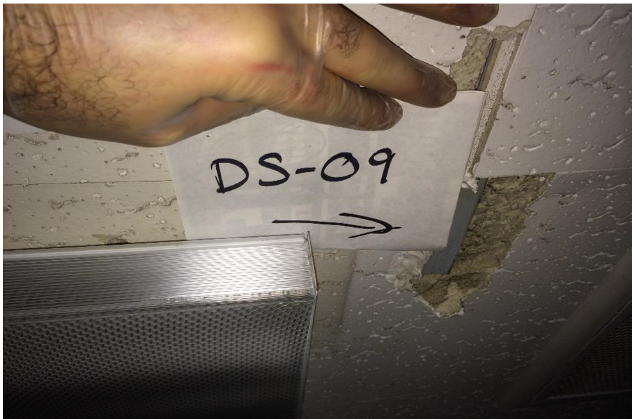
Plate 34: Laboratory analyses detected 3% chrysotile asbestos and 3% amosite asbestos within suspended ceiling tile sample DS-09 collected from the Dormitory Building upstairs computer room.
