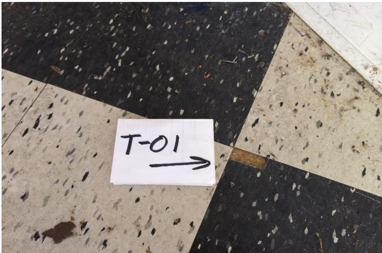
Plate 52: Laboratory analyses did not detect asbestos minerals within the black floor tile from sample TS-01 but did detect 5% chrysotile asbestos in the mastic from sample TS-01 collected from the Theatre Building lobby area.
