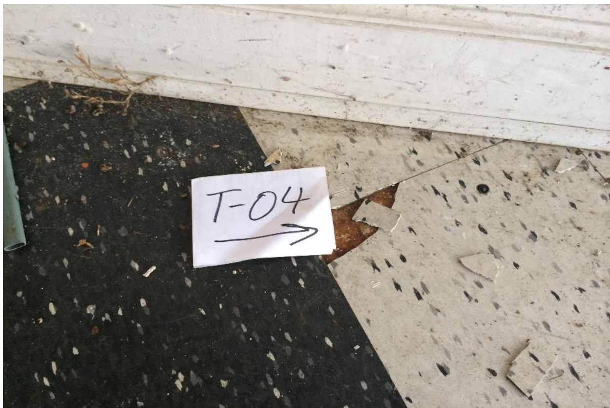
Plate 55: Laboratory analyses did not detect asbestos minerals within the white floor tile from sample TS-04 but did detect 5% chrysotile asbestos in the mastic from sample TS-04 collected from the Theatre Building lobby area.
