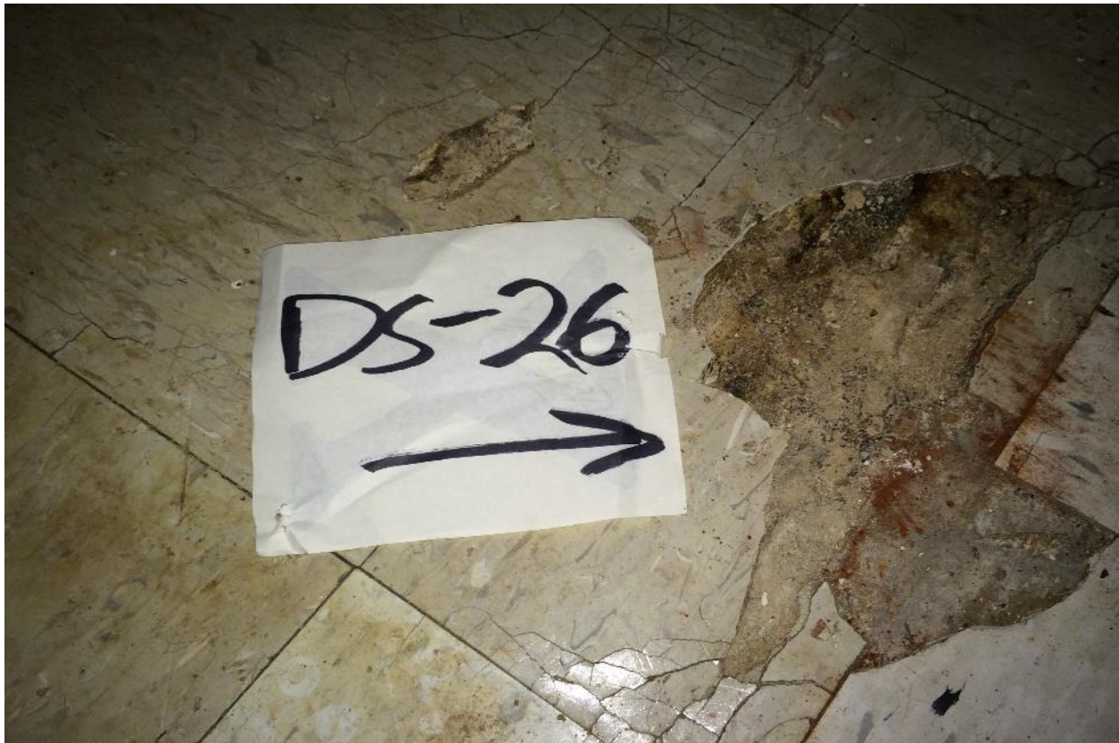
Plate 51: Laboratory analyses did not detect asbestos minerals within the black floor tile or mastic sample DS-26 collected from the Dormitory Building downstairs east miscellaneous rooms.
