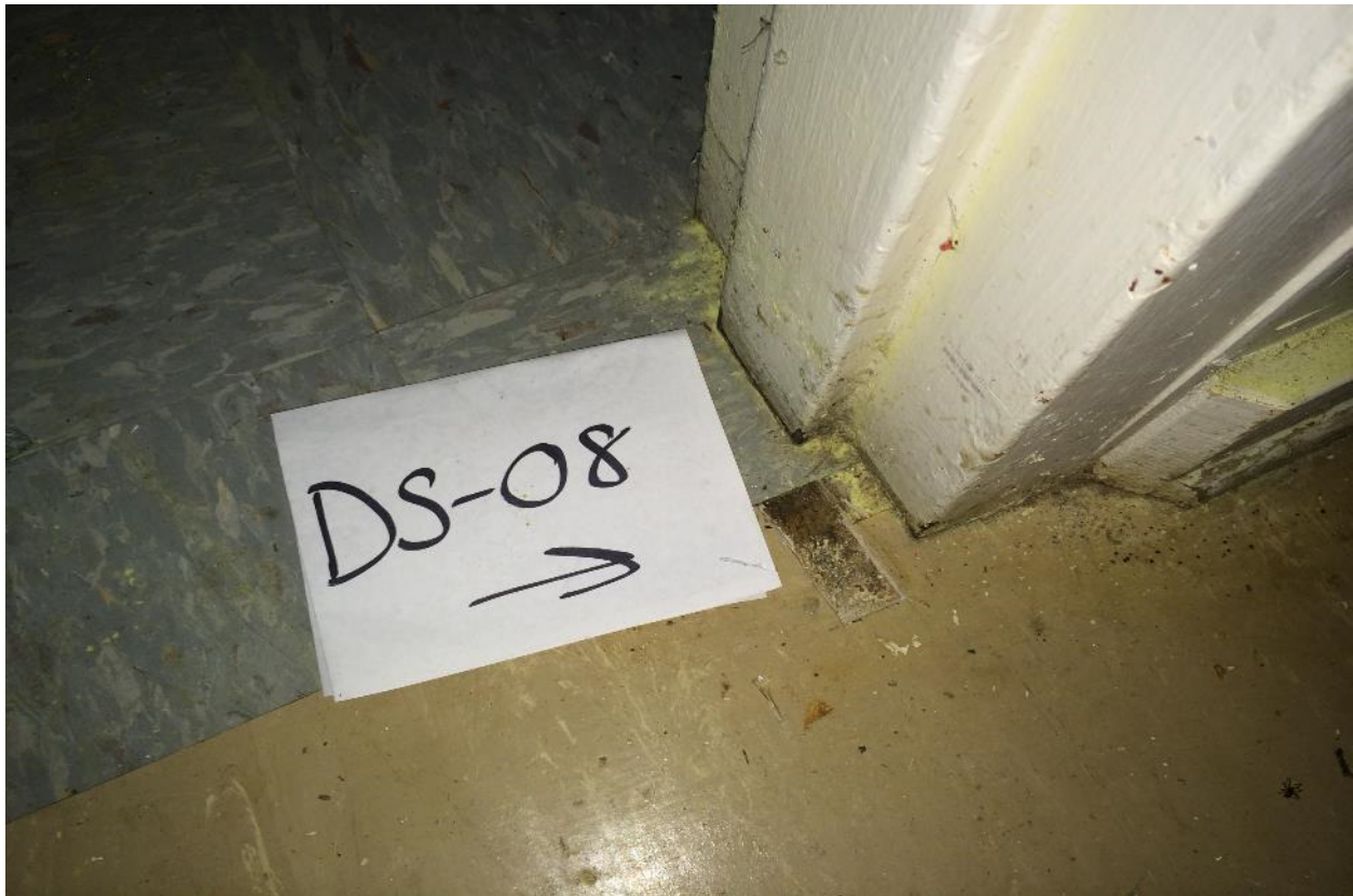
Plate 33: Laboratory analyses did not detect asbestos minerals within the beige floor tile or mastic sample DS-08 collected from the Dormitory Building upstairs hallway.
