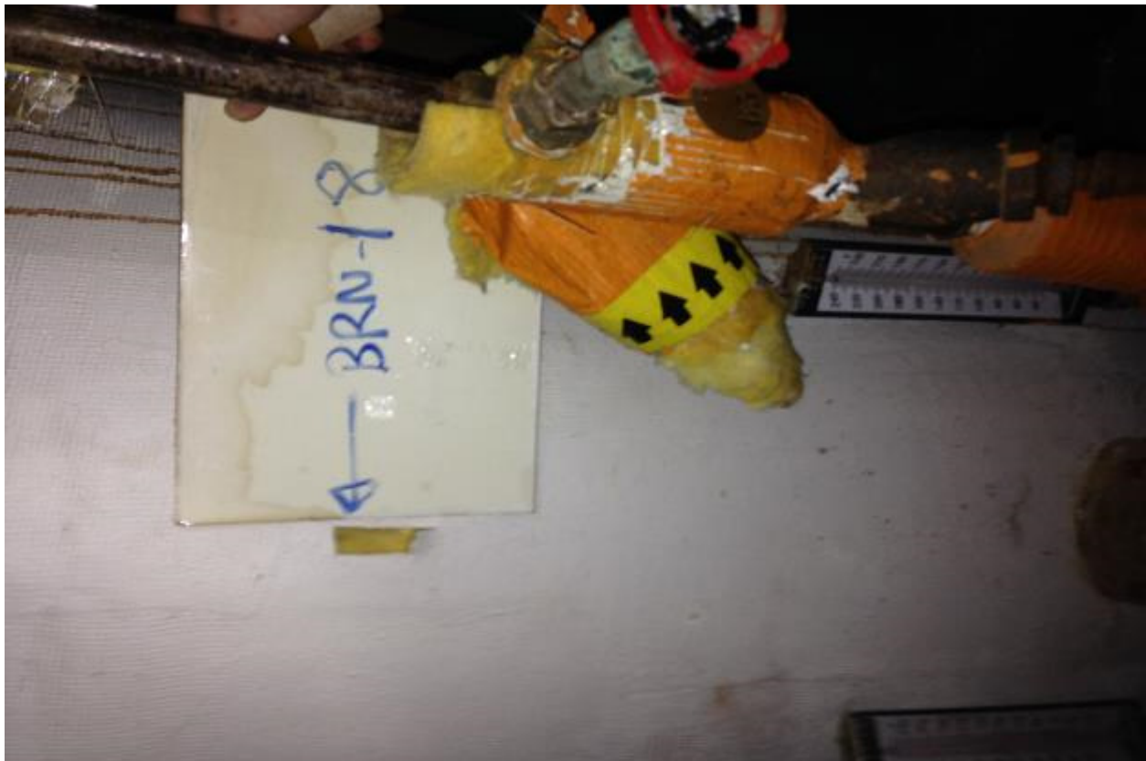
Plate 18: Laboratory analyses did not detect asbestos minerals within Boiler Wrap sample BRN-18 collected from the North Administrative Building mechanical room.
