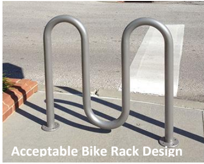
Figure 12-1A: Acceptable Bike Rack Designs
