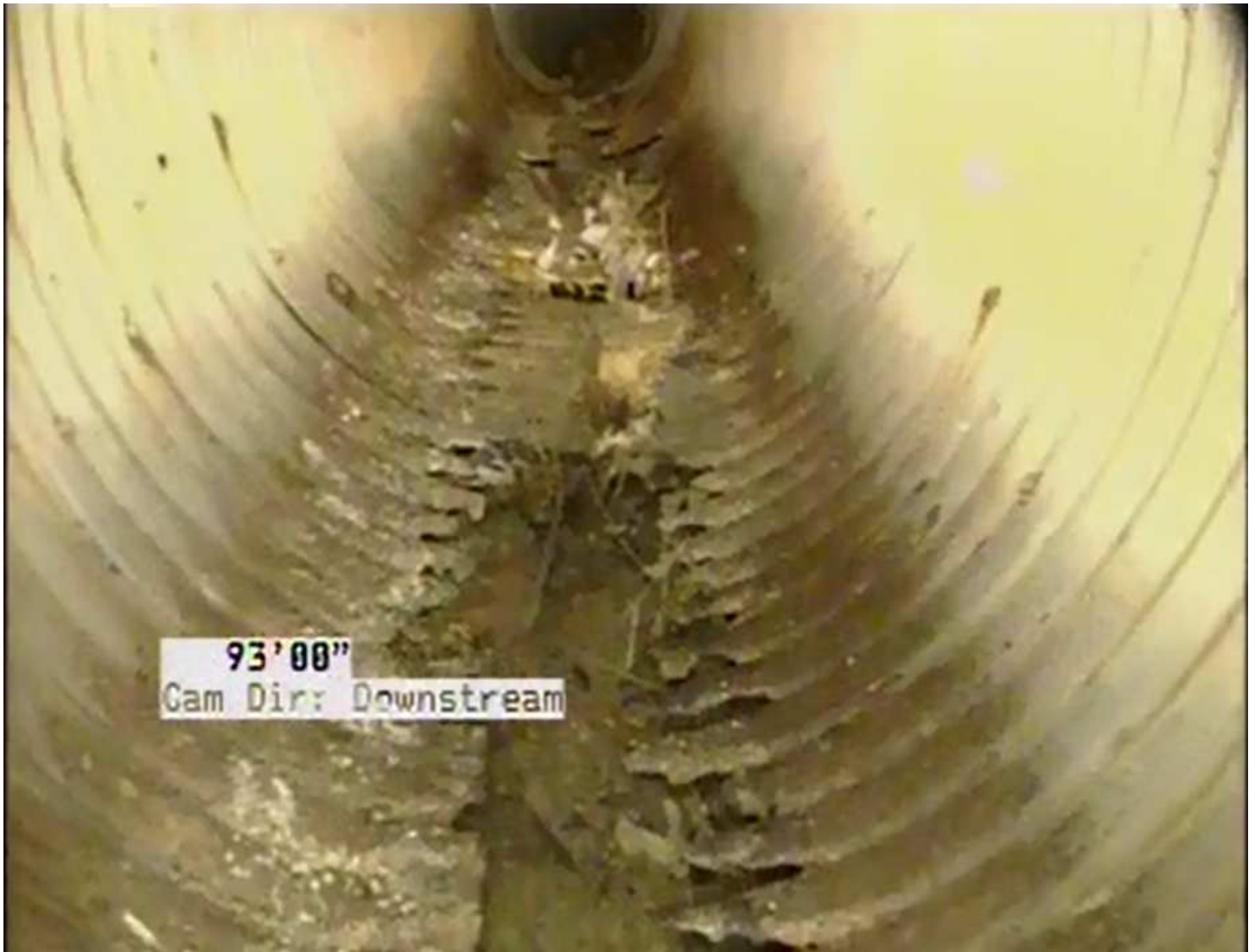
Deteriorated portions of 30" Corrugated Metal Pipe
