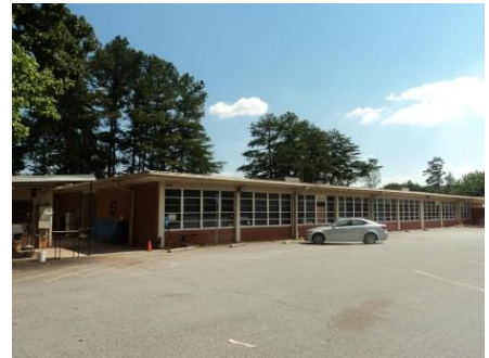
Education Center Rear Classroom Wing
