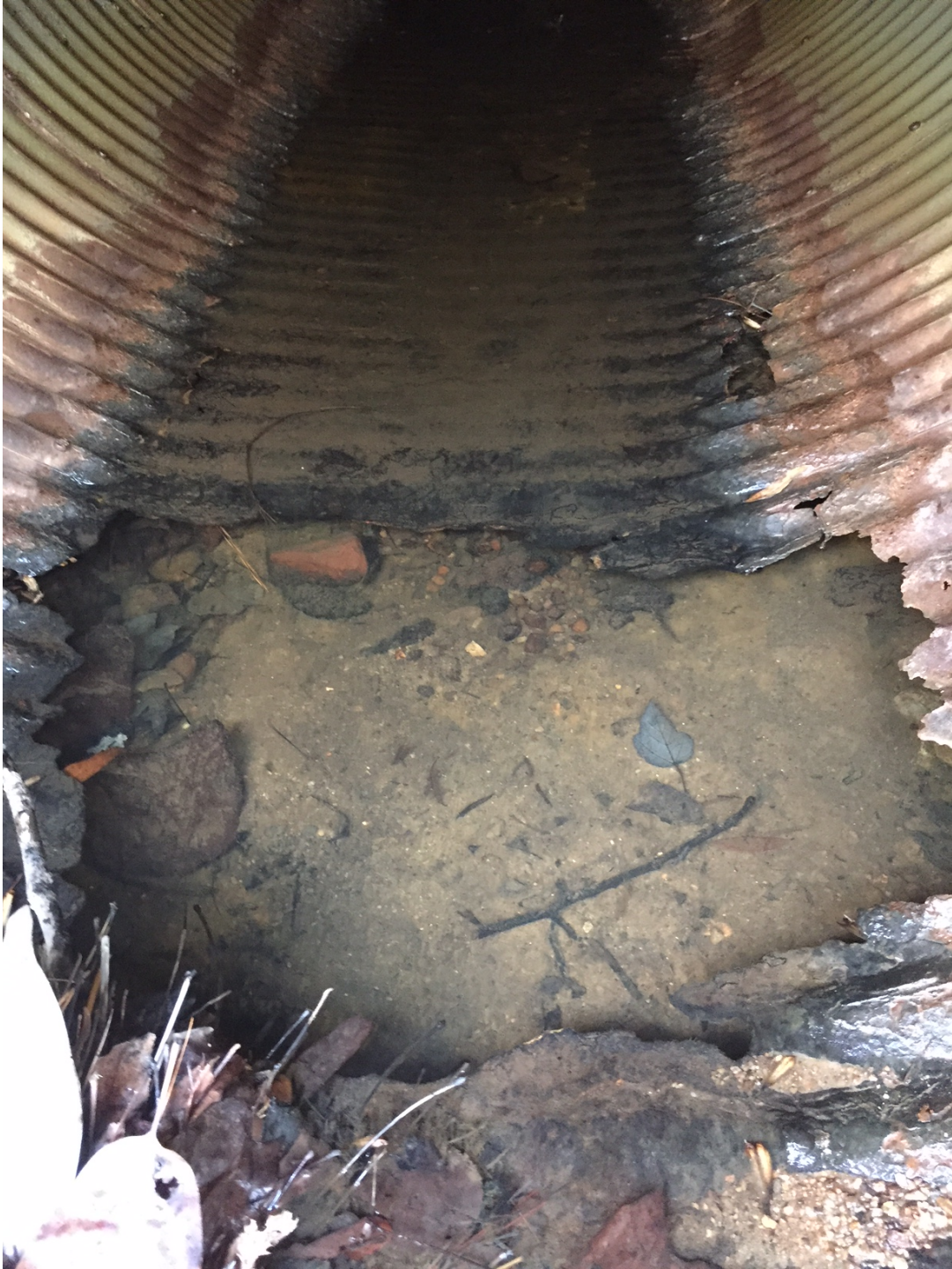
Missing invert in portions of 60" culvert
