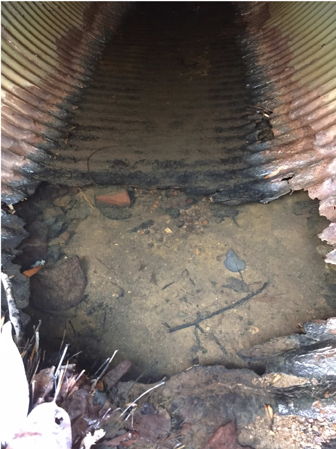
Missing invert in portions of 60" culvert
