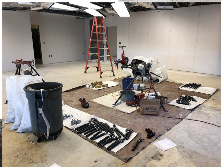
New Fire Sprinkler System being installed in entire building
