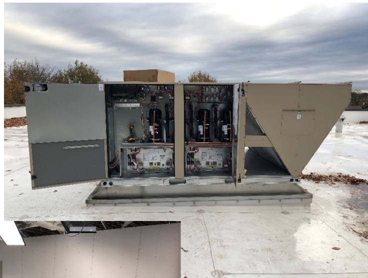
New Roof Top HVAC Unit Installed to service 2 nd floor
