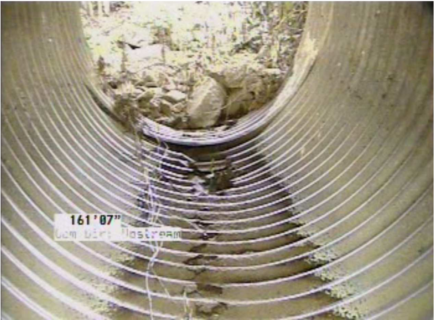
Rusting and Pipe Deterioration due to age
