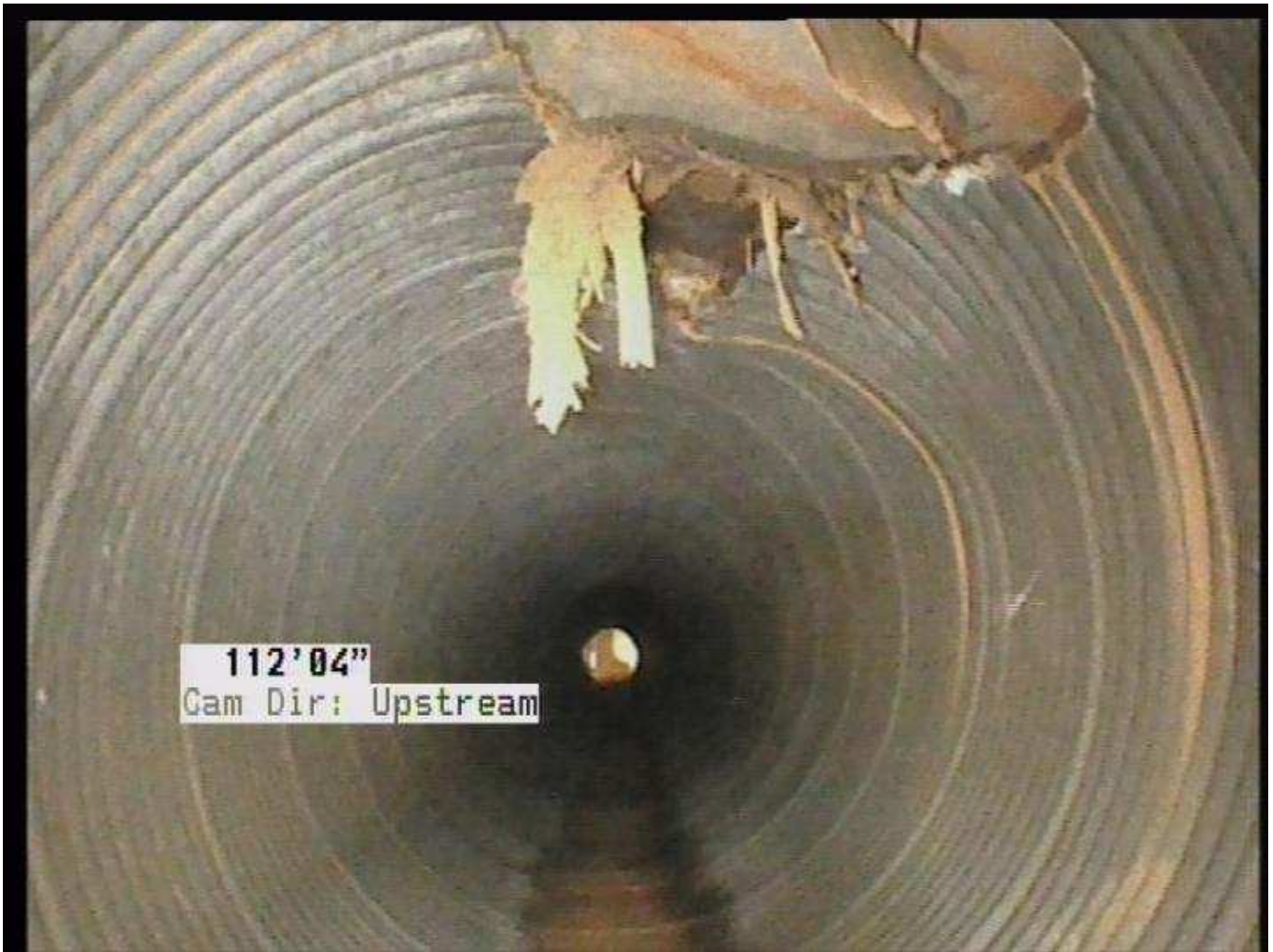
Pipe Damage From Original Construction
