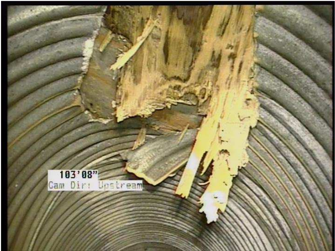
Pipe Damage From Original Construction
