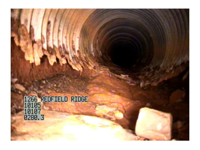
TOTAL INVERT FAILURE IN PIPE
