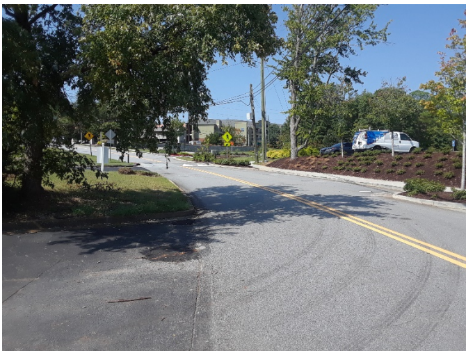
SOUTHWEST ALONG PERNOSHAL COURT
