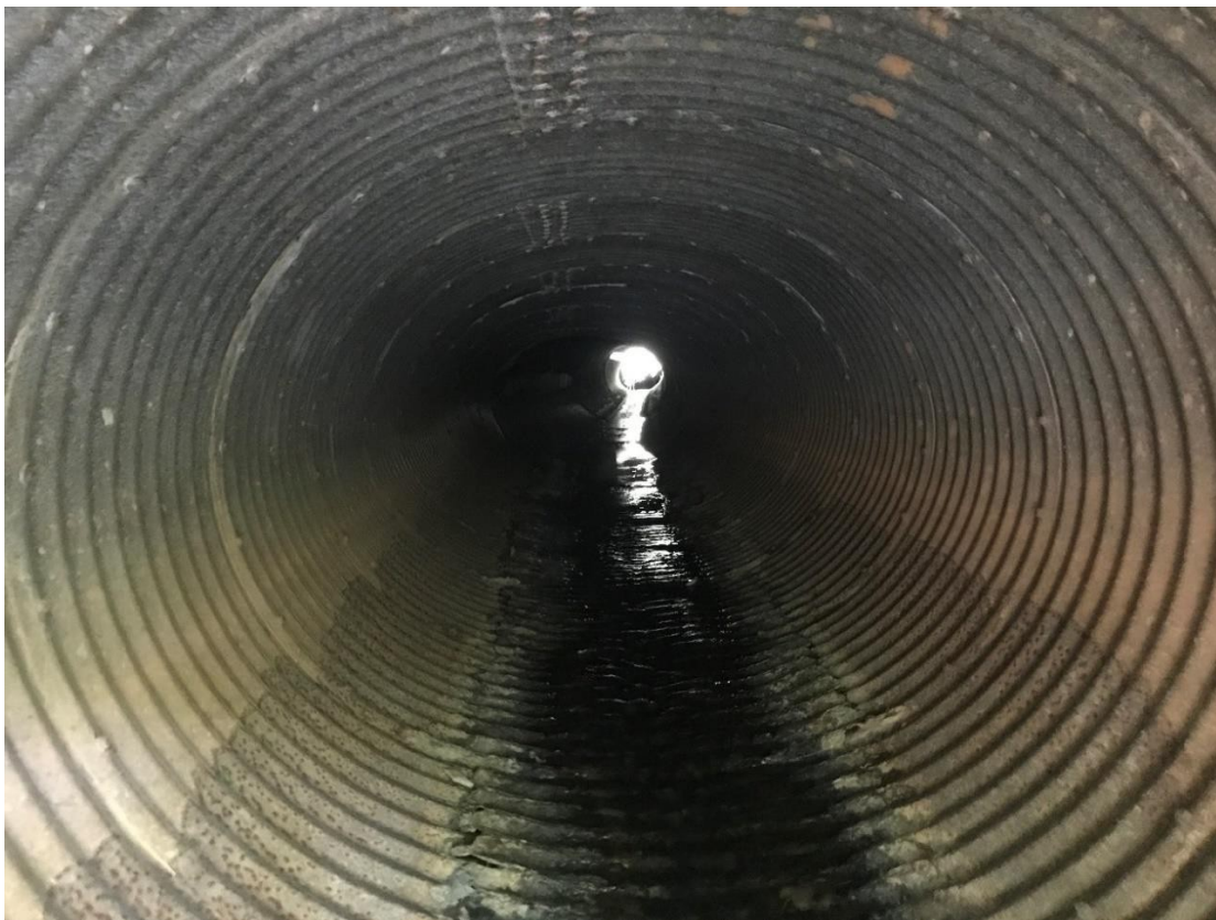
Deformed metal pipe with invert corrosion & visible holes
