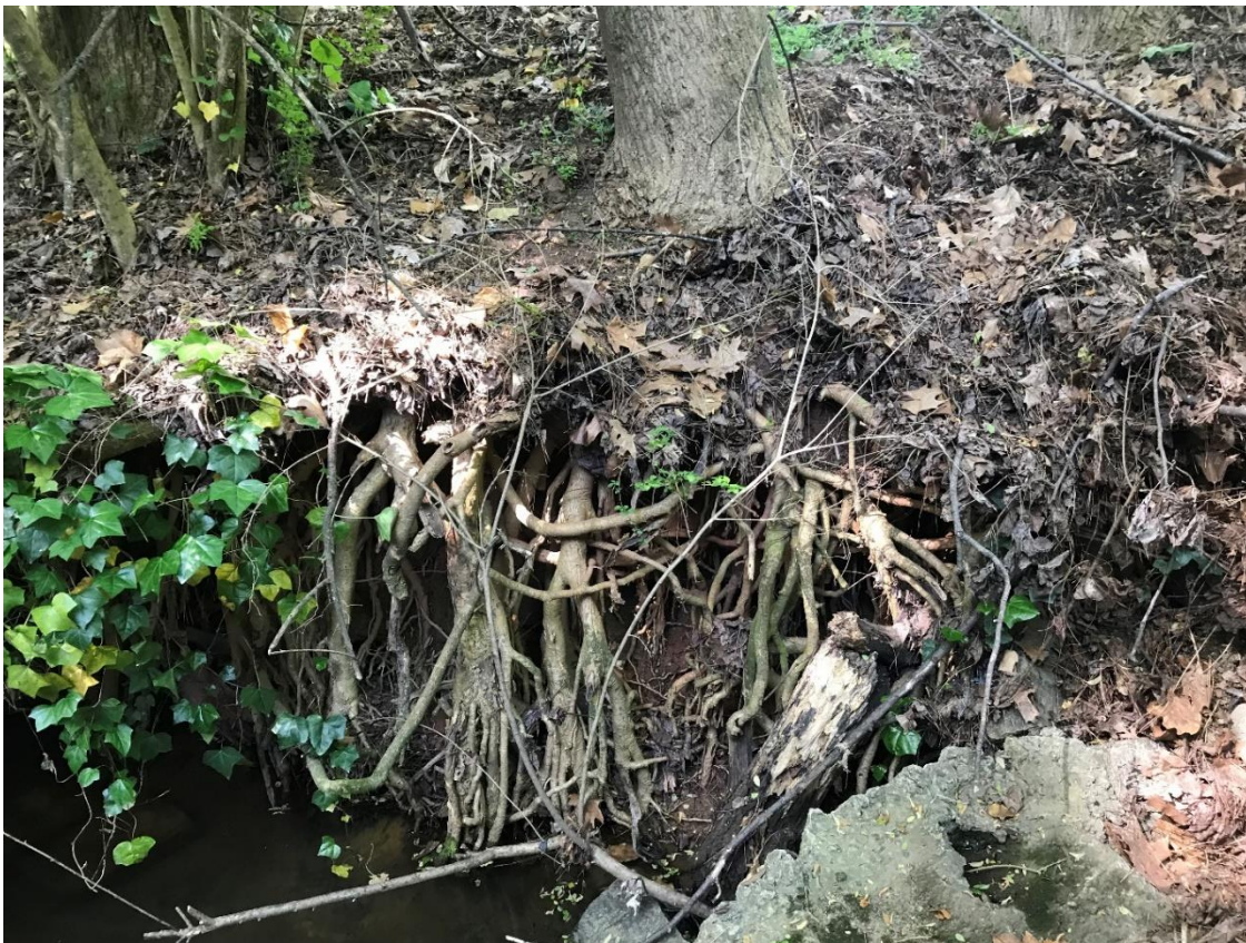
Embankment scour exposing tree roots
