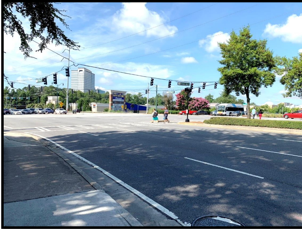
Photograph 1 – Ashford Dunwoody Road Facing South at Ravinia Parkway
