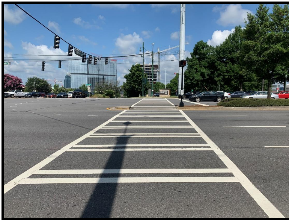
Photograph 3 – Two-Stage Pedestrian Crossing of Ashford Dunwoody on North Side of Ravinia
