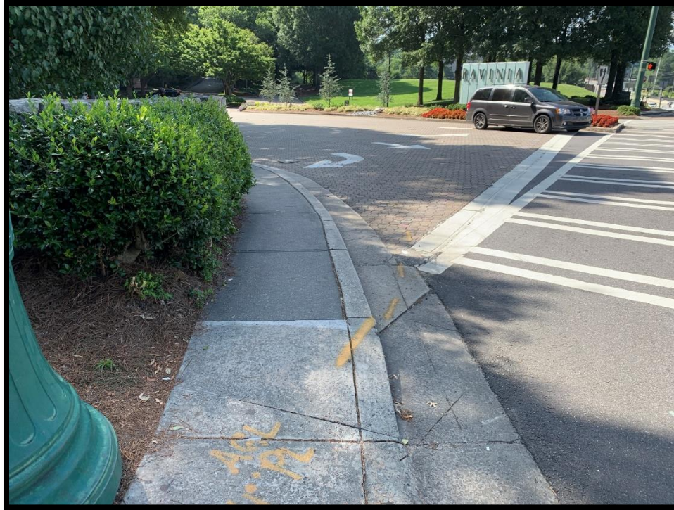
Photograph 2 – Narrow Sidewalk and Lack of Lane Striping in Northeast Corner of Ashford Dunwoody at Ravinia
