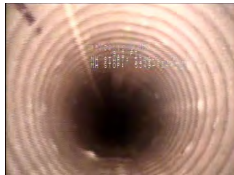
Cured In Place Pipe (CIPP) repair on Mt Vernon Road (2019)
