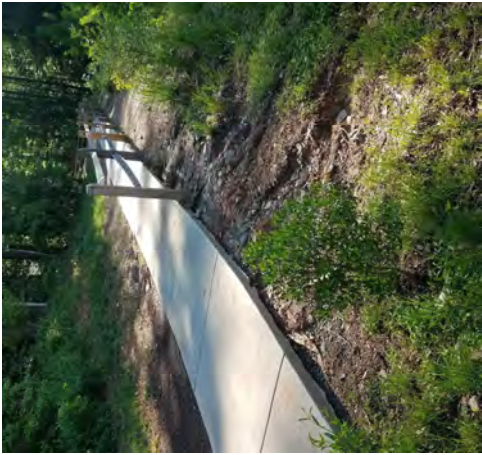
Stormwater runoff is undercutting the existing sidewalk north of the pond, creating a safety hazard.
