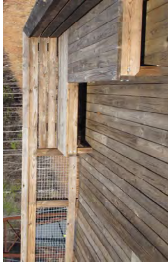
Constructing a hexagonal deck (inspired by the honeycomb) off of the existing eco-classroom provides additional amenity space while contributing to resolving the significant stormwater runoff issues in the area.
