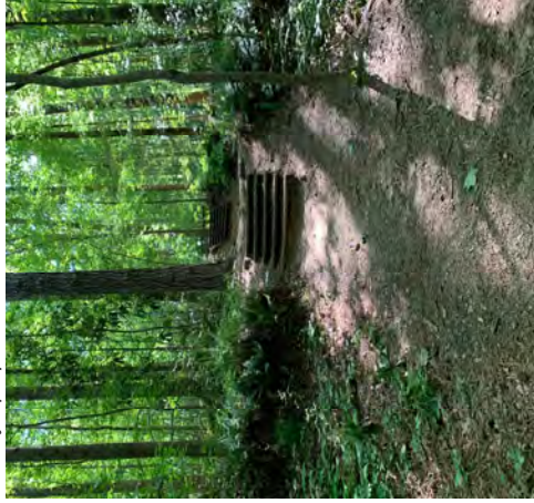
Stormwater runoff issues caused significant erosion and exposed large amounts of tree roots. This is a tripping hazard for people and causes stress on the tree.
