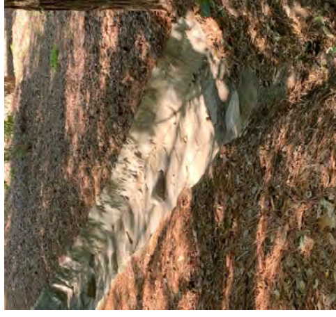
Existing concrete drainage swale is full of debris, reducing its functionality.
