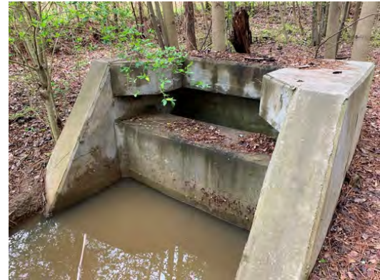
EXISTING BAFFLED INLET
