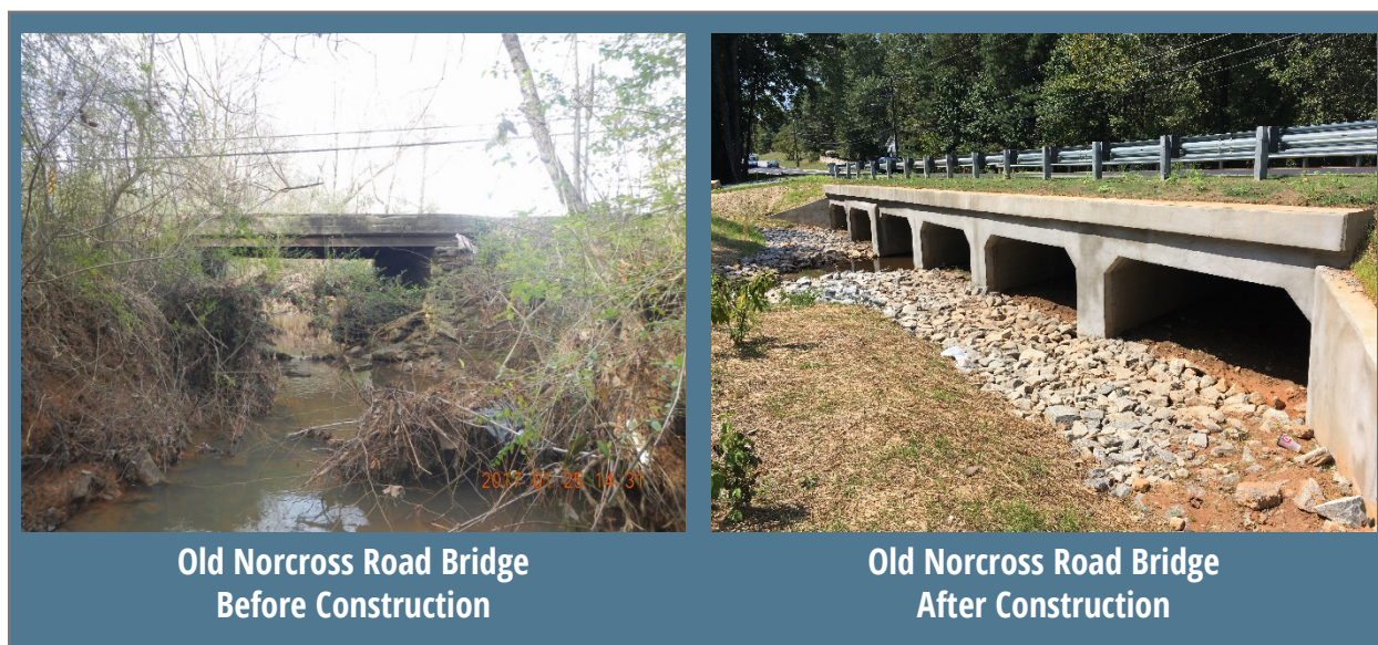
FIGURE 3: Dewberry developed the design, construction documents, and specifications, and provided permitting and bid assistance to replace the existing 19-foot span bridge on Old Norcross Road to address safety and hydraulic capacity deficiencies. Dewberry also provided construction management services, and construction was completed within budget.
