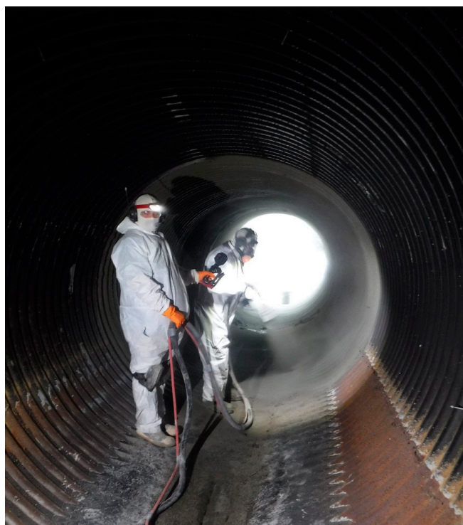
FIGURE 5: Application of CCCP for a design project completed by Dewberry for Gwinnett County. CCCP was selected to extend the useful lifespan of the existing CMP and increase the resilience of the stormwater system.
