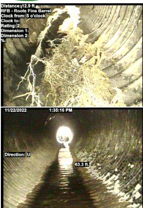
Severe Corrosion, Joint Separation, and Root Infiltration
