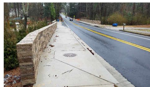
Fayette County, Stormwater Services
