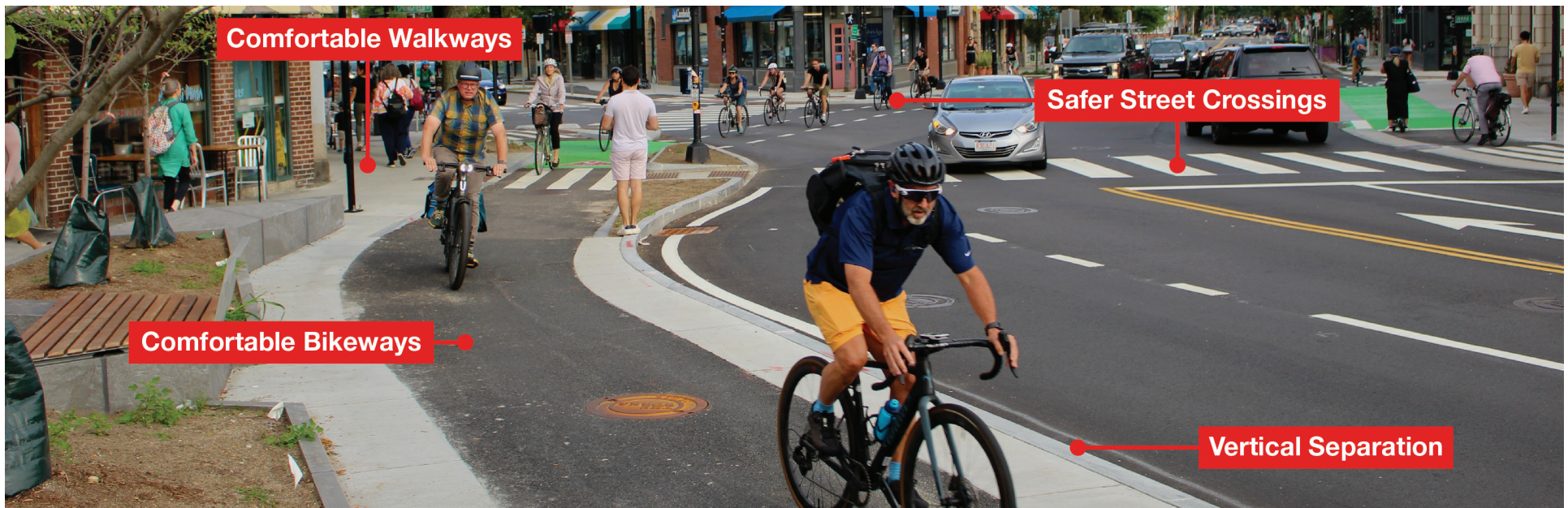
Complete Street in Cambridge, MA. Source: Toole Design Group
