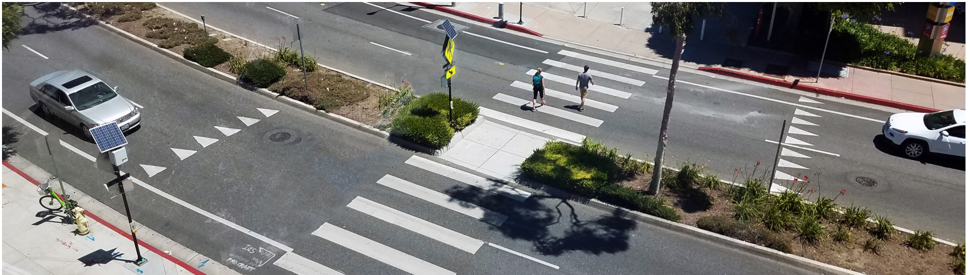
RRFB and median island in West Hollywood, CA Source: Toole Design Group
