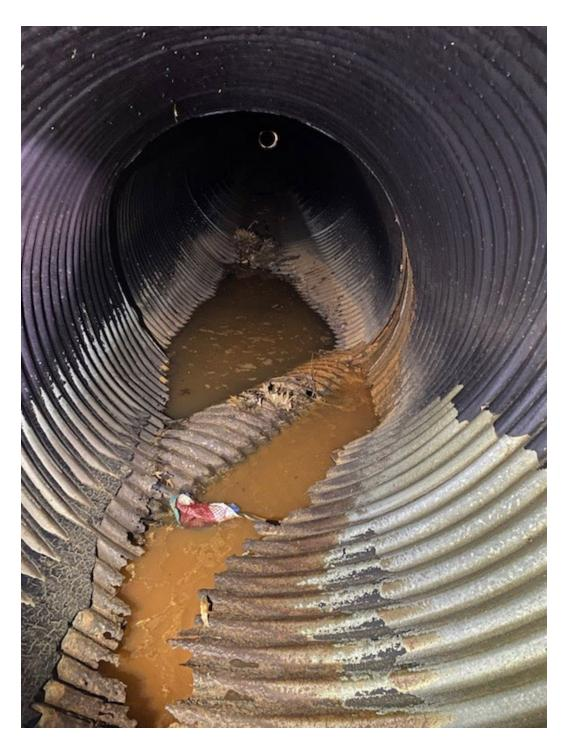
**Severe Invert Corrosion** Joint Separation Water Sagging
