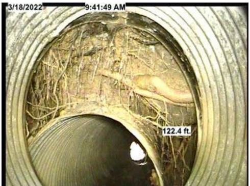
**Invert Corrosion With Large Holes Major Joint Separation**
