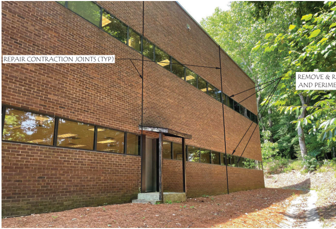
2 ELEVATION - PARTIAL NORTH WALL ELEVATION REPAIRS SCALE: NOT TO SCALE
