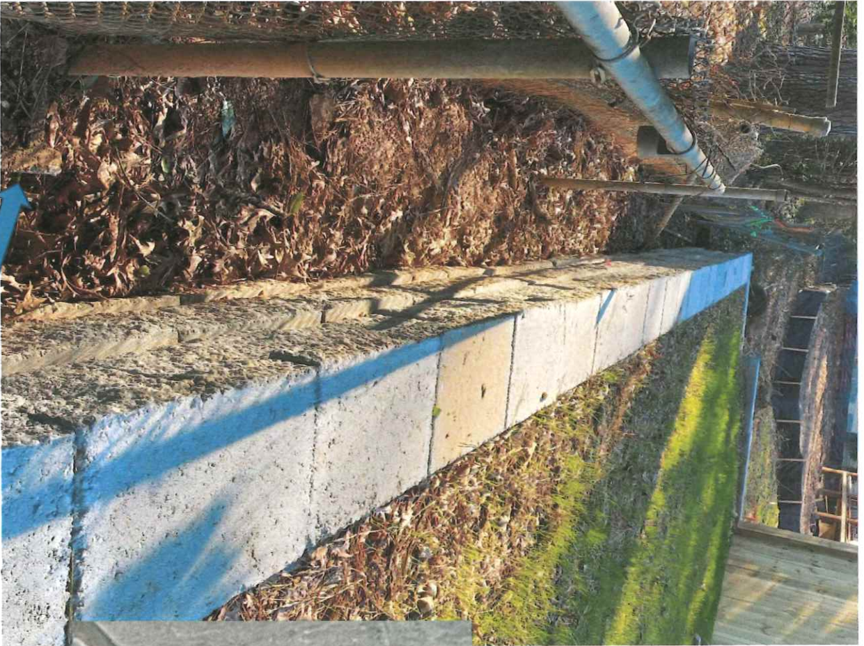
Back of L-shaped Retaining Wall.
