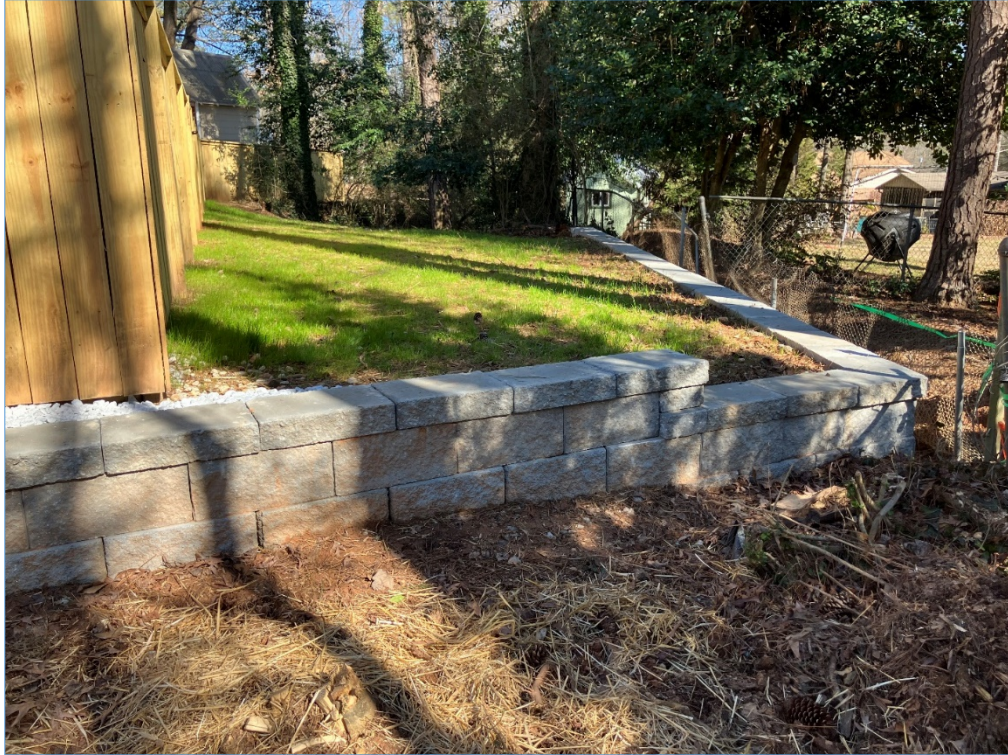
The retaining wall.
