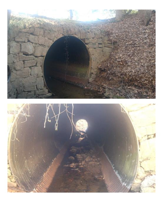
Stone Headwall -w- moderate grout deterioration **Invert Corrosion With Visible Holes Major Joint Separation**
