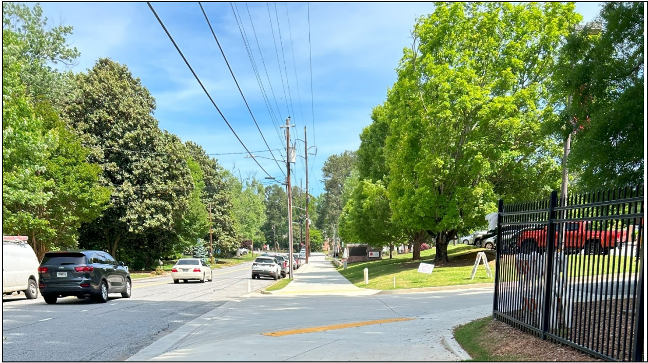
Phase I Path completed, July 2023 to Vanderlyn Drive
