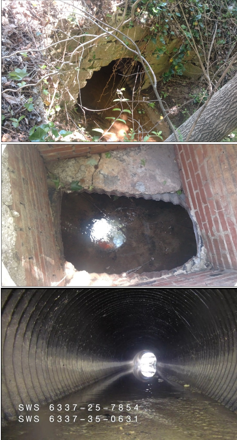
Corrosion, Joint Separation
