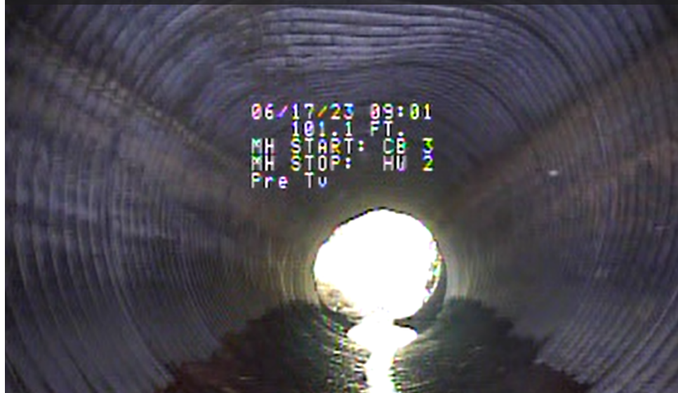
Deformation, Joint Separation
