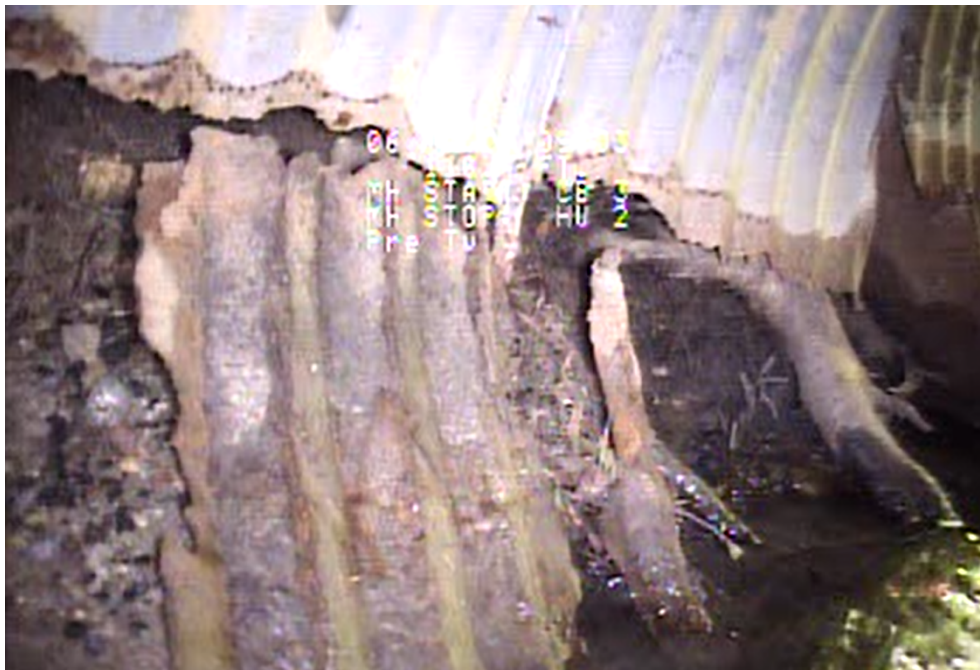
Severe Corrosion, Holes
