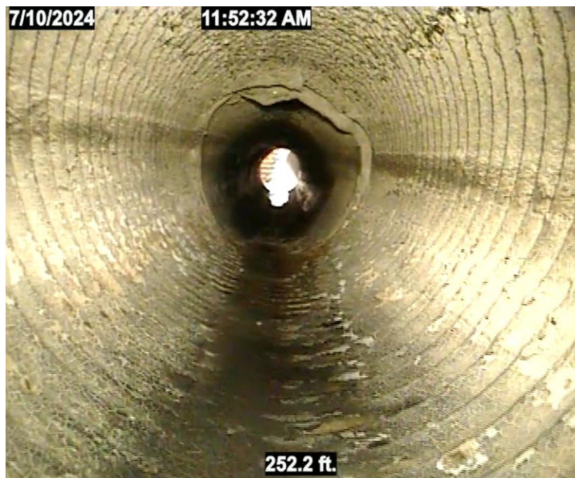
Deformations and Joint Offsets. Bituminous Coating worn away with visible rusting of invert.
