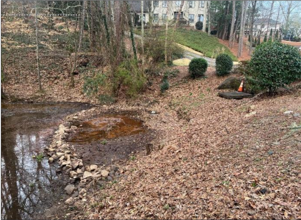
View of Existing Outlet Control Retrofit covered by debris. Orange cone sitting on top of the overflow grate inlet.
