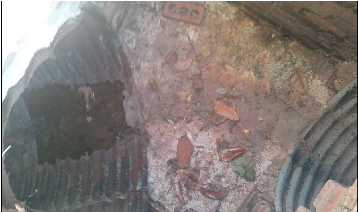
Large hole in bottom of pipe. Supporting soils undermined.
