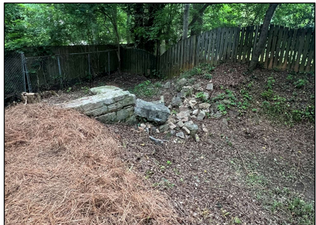
Breached rubble wall (5/19/2025)
