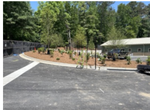
Brook Run Maintenance Facility
