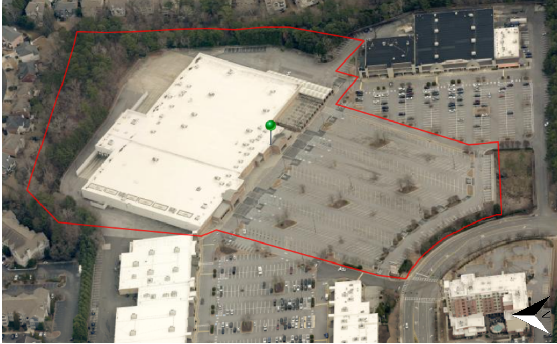
Fig. 1, Aerial view of subject site
