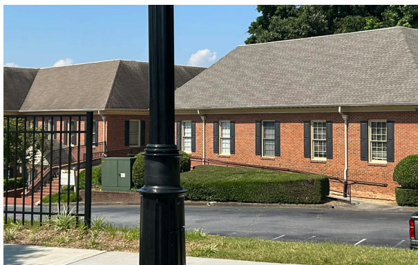
Large office development lacking connectivity
