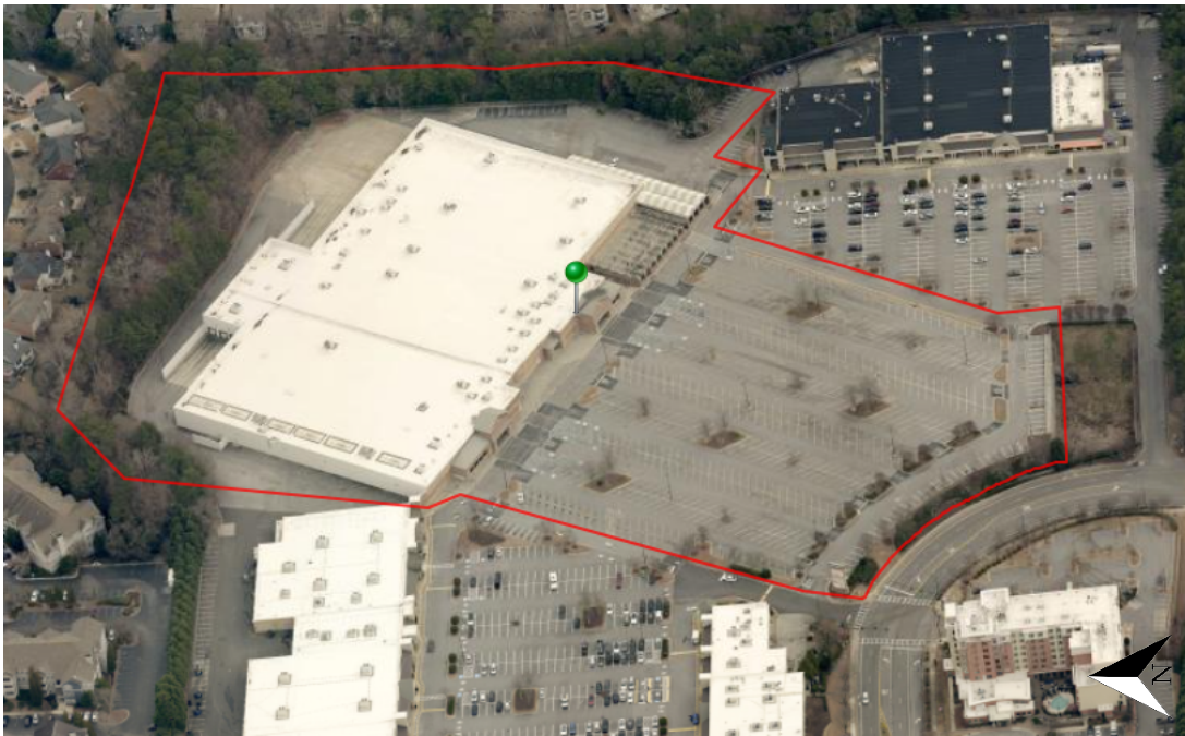
Fig. 1, Aerial view of subject site
