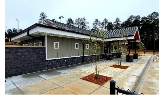
Tennis Center Restrooms
