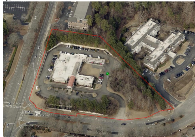
Aerial view of property, looking north
