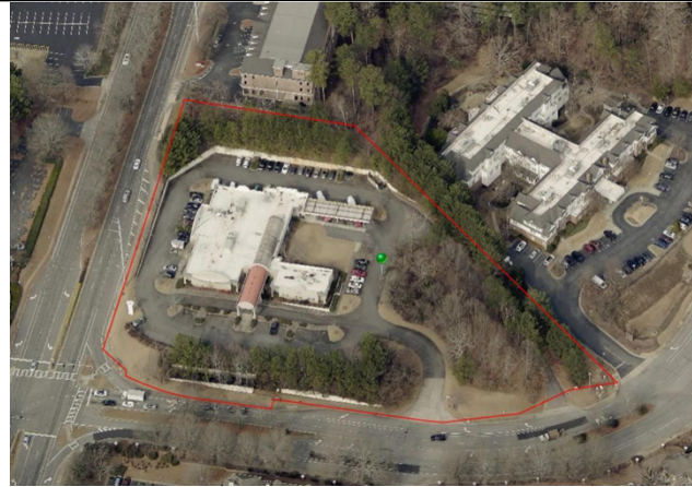
Aerial view of property, looking north
