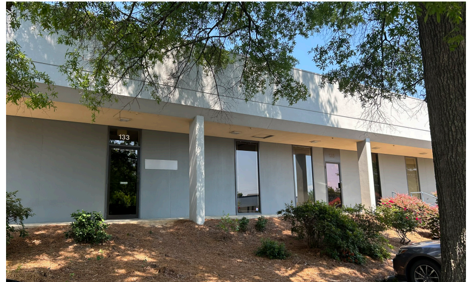
Existing Conditions at Dunwoody Park & Lofts
