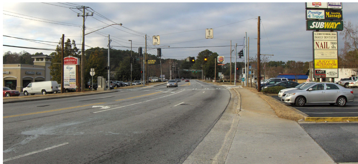
Before - Chamblee Dunwoody Road looking north
