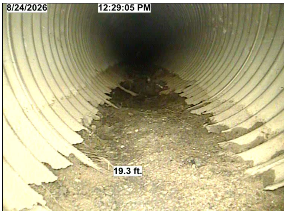
CCTV – Upstream Viewing Direction, Measured 19.3 LF from outlet.
