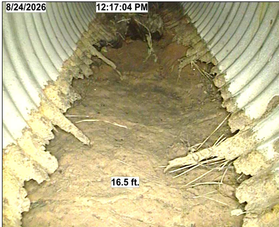
CCTV – Downstream Viewing Direction, Measured 16.5 LF from Catch Basin.
